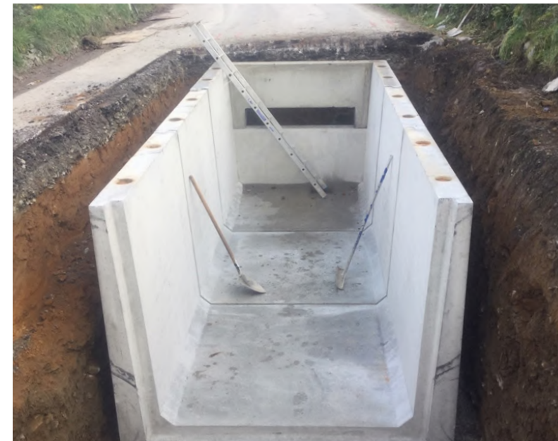
Figure 3: A typical jointing bay where cables are connected
