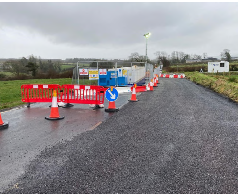
Figure 5: A typical passing bay in operation during cable jointing
