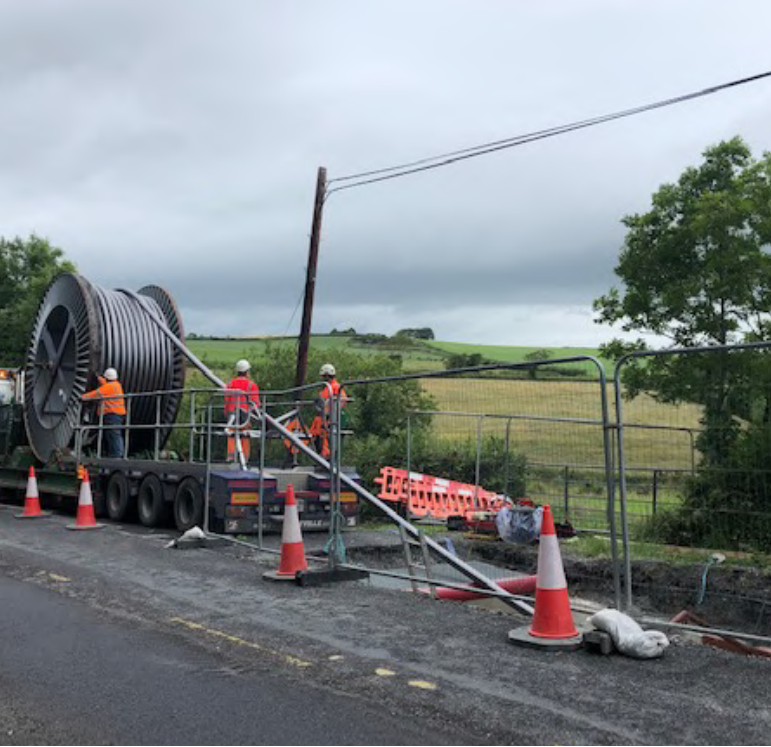
Figure 4: Cables being pulled into the ducts and jointing bay
