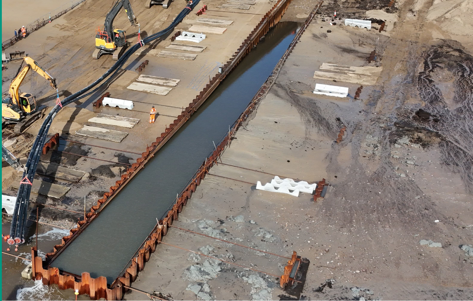
Ducting pipes being lifted synchronously to the cofferdam (trench) at Claycastle Beach, March 2025.
