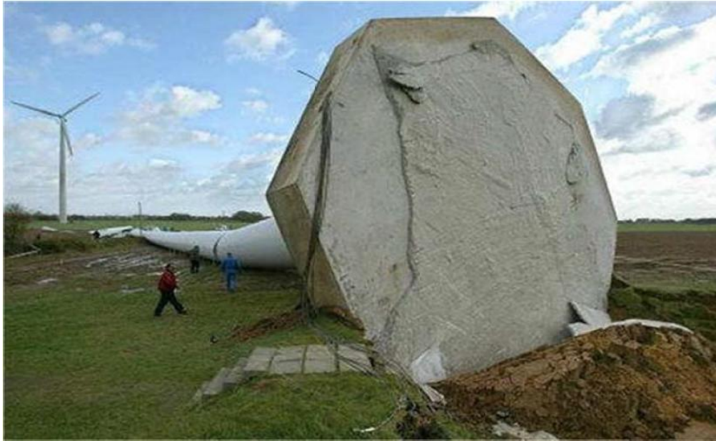
Figure 3 Fallen turbine
