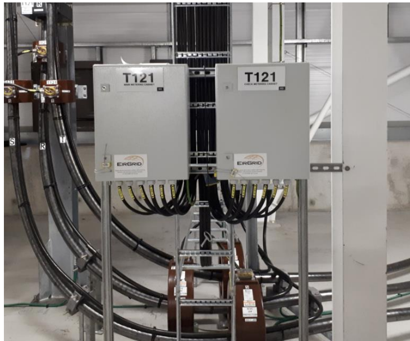
Picture 1: Metering marshalling kiosk
