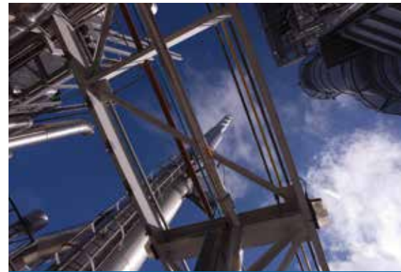
Tynagh Power Station.
