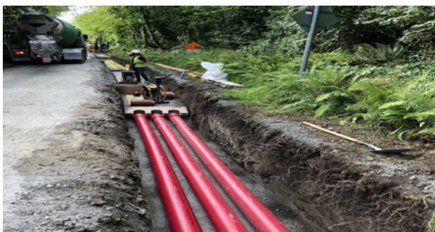
Figure 5: A typical cable duct installation in the road
