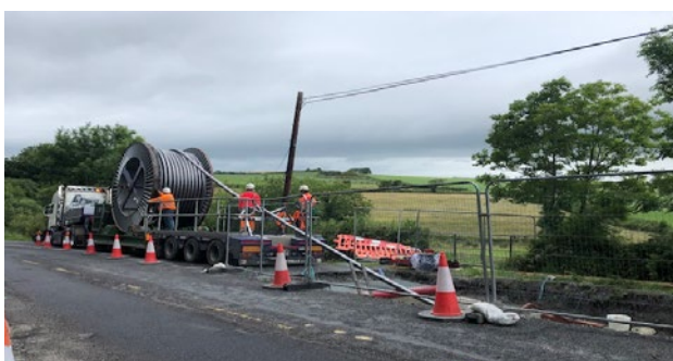
Figure 7: Cables being pulled into the ducts and jointing bay
