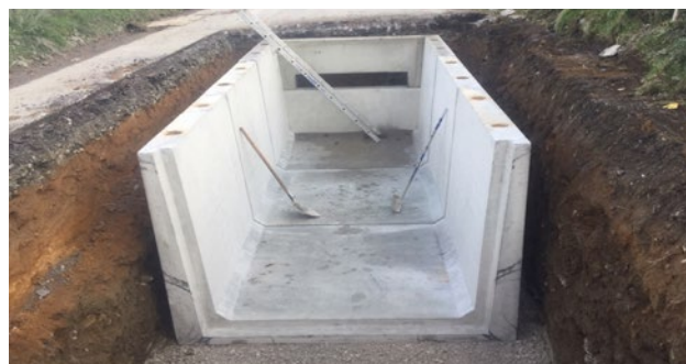
Figure 6: A typical jointing bay where cables are connected
