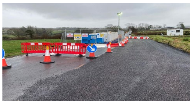
Figure 8: A typical passing bay in operation during cable jointing
