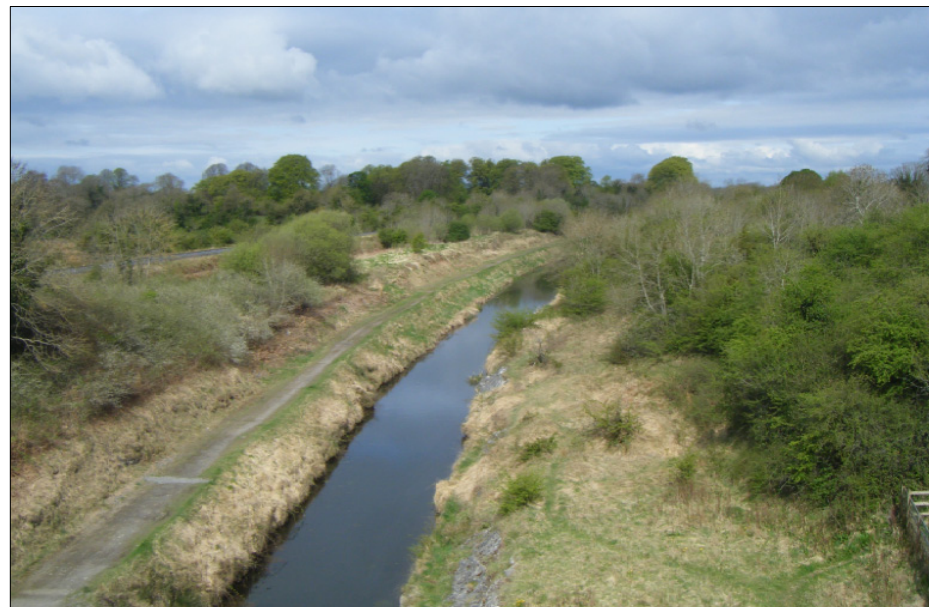
Plate 4: Royal Canal at Boardstown
