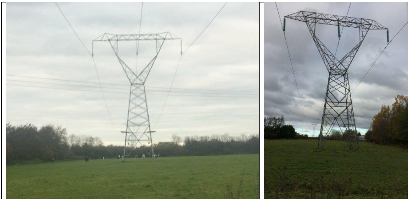
Figure 3.8. Single circuit 220kV Suspension Towers (Maynooth-Gorman)
