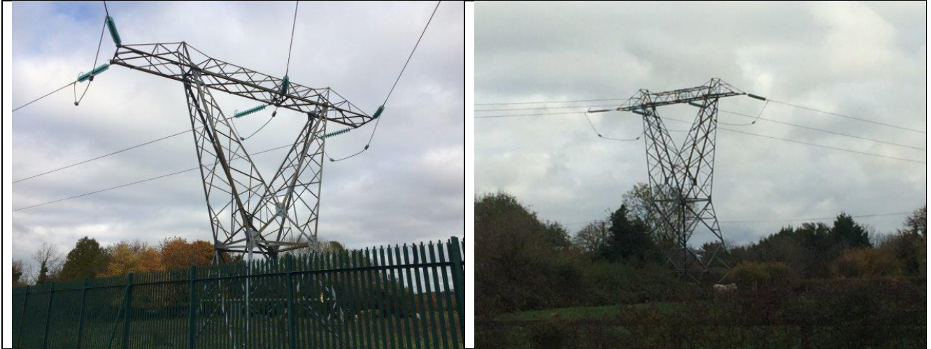
Figure 3.9. Single Circuit 220kV Section / Angle Towers (Dunstown-Maynooth)
