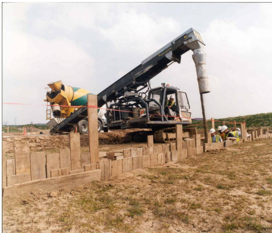
Figure 11 Delivery of CBS to the Cable Trench
