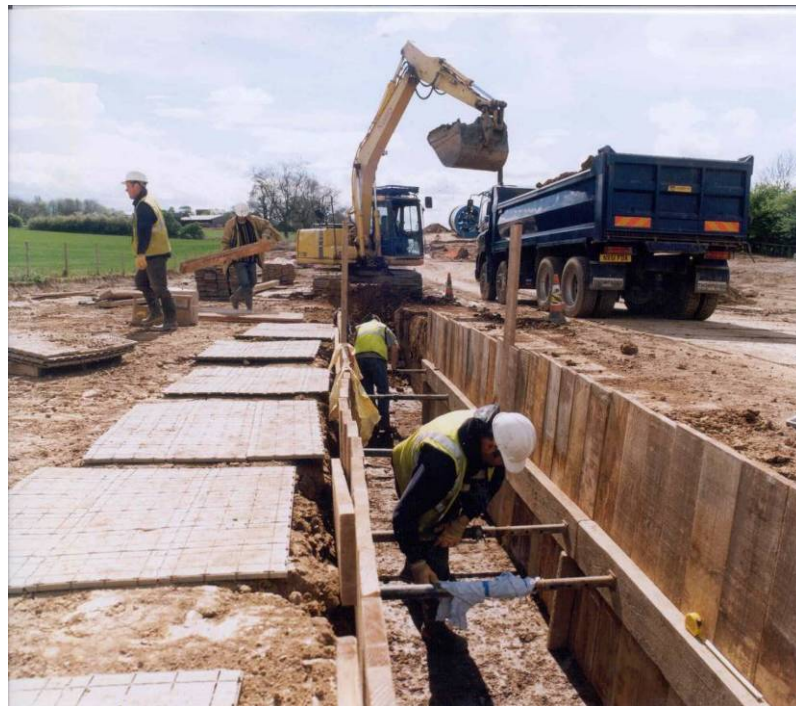
Figure 6 A Close Timbered Cable Trench
