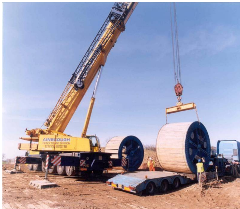
Figure 9 Offloading Cable Drums
