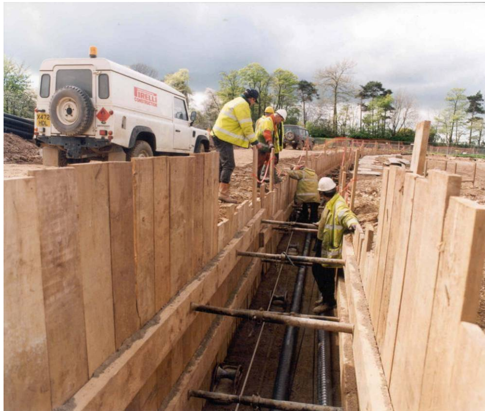
Figure 10 Cable installation in an Open Cut Trench
