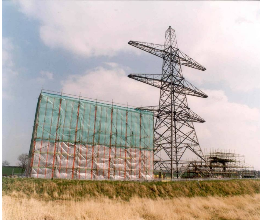
Figure 12 Weatherproof Sheeted Enclosure for Cable Termination Assembly
