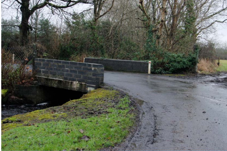
Road B: Bridge followed by a sharp bend
