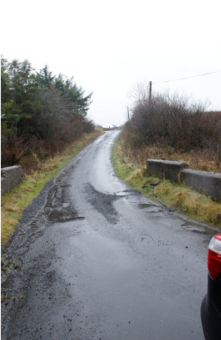
Road A: Example of steep slope from the bridge
