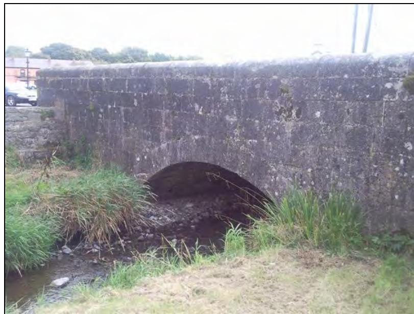
Figure 5.14 The stone bridge cover entering Timahoe village
