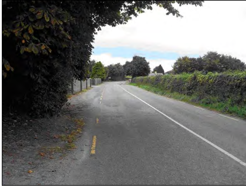
Figure 5.1 The seven metre wide R432 at Ballyragget 110 kV Station
