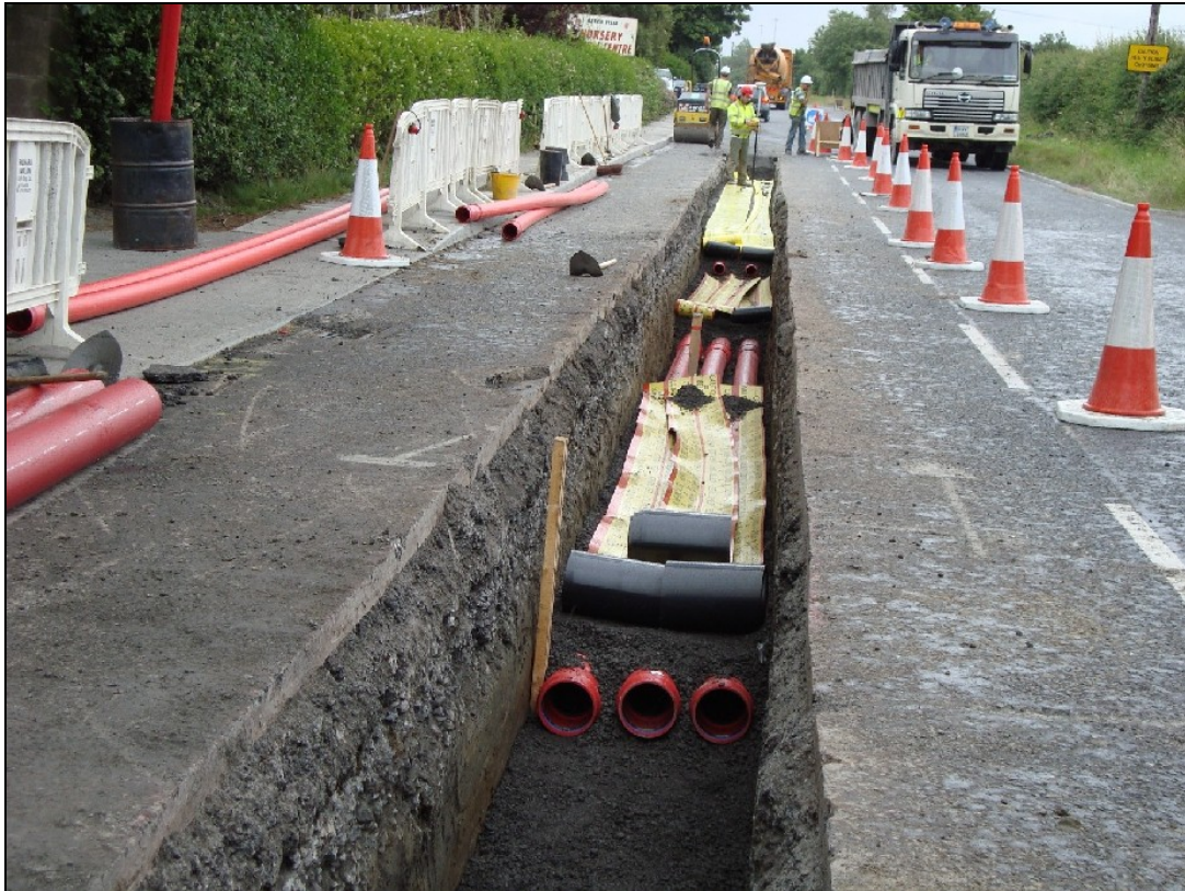
Figures 3.2 – 3.4 Construction of Underground Cables
