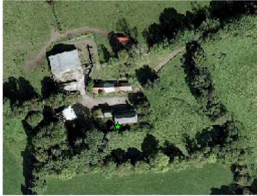
Figure 8: Crossmahon House, an example of a protected structure (Green Star)
