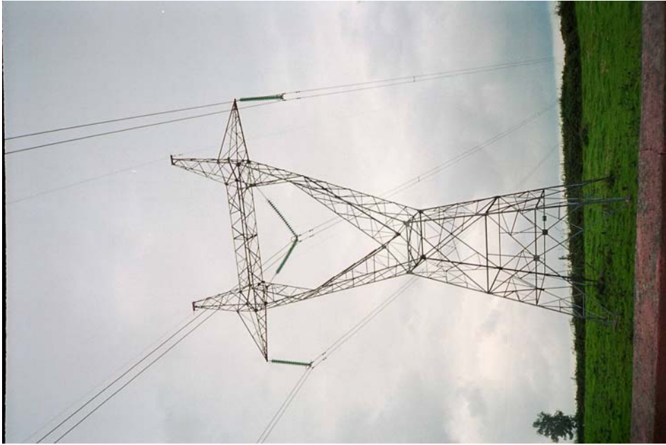
Indicative 400kV Single Circuit Intermediate Tower
