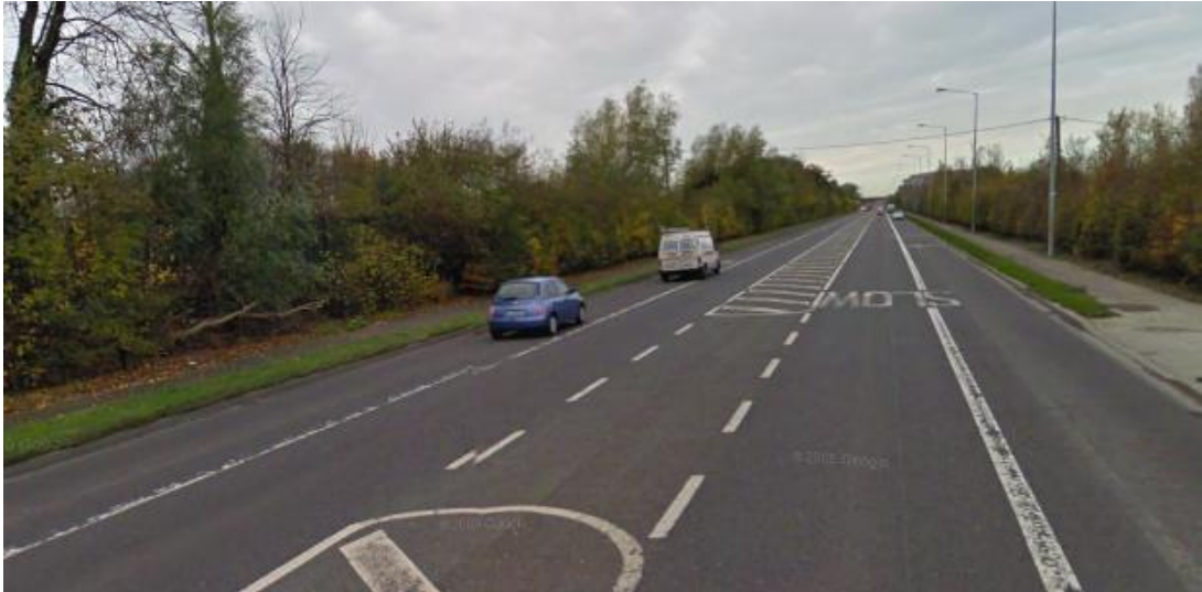
Fig 4.1: N32 National Route Looking West
