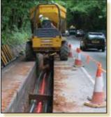
The circuit between the converter station and the landfall point will be by underground cable installed in ducts under the road network, which will be fully re-instated. The total length of this circuit is expected to be between 30 – 40 km.
