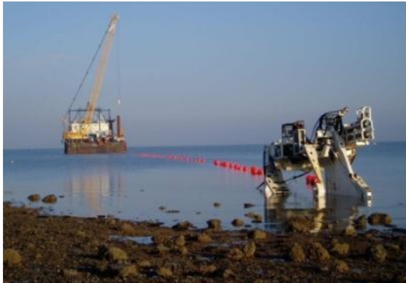
Figure A-3: Cable lay barge offshore end with plough on the beach
