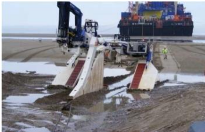
Figure A-2: Cable plough on beach
