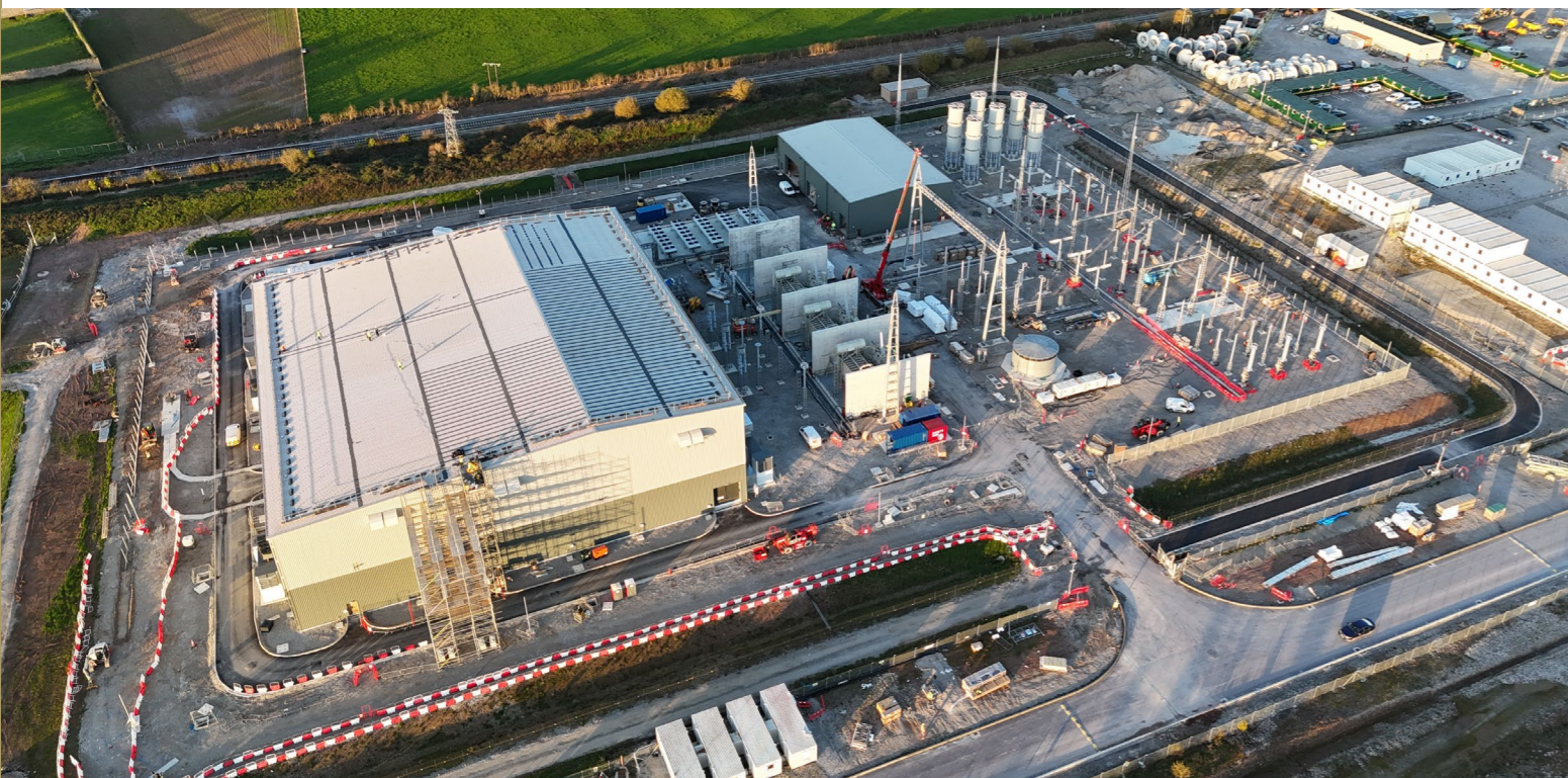
Converter station civil works are nearing completion.
