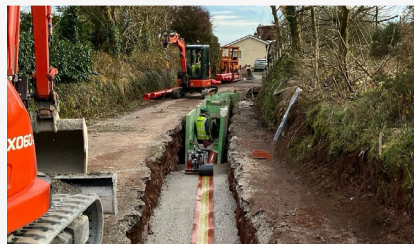
Trenching and ducting works progressing.
