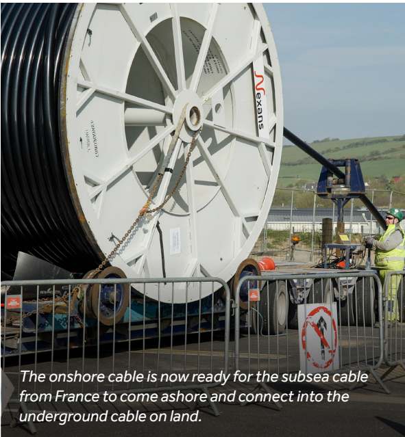
The final onshore cable installation was completed at Claycastle Beach, Youghal.
