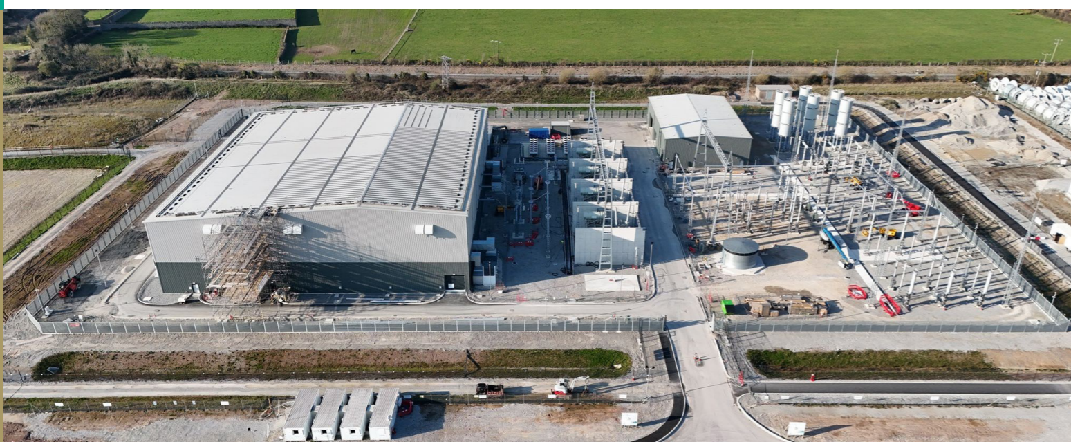
Converter station site, Ballyadam.
