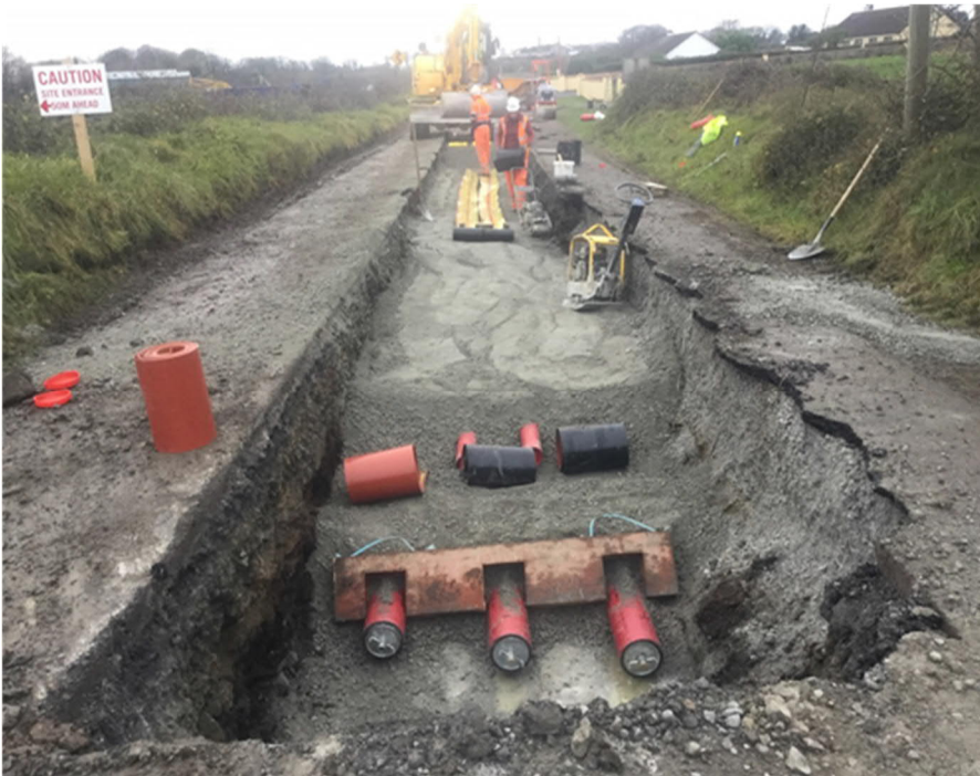
Figure 15: HVAC Cable Trench in Road (showing one cable per phase)
