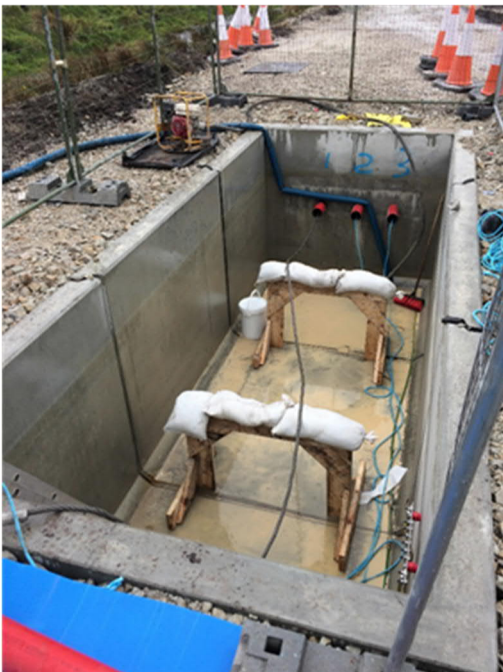
Figure 16: Example of a HVAC joint chamber in preparation for pulling of cable
