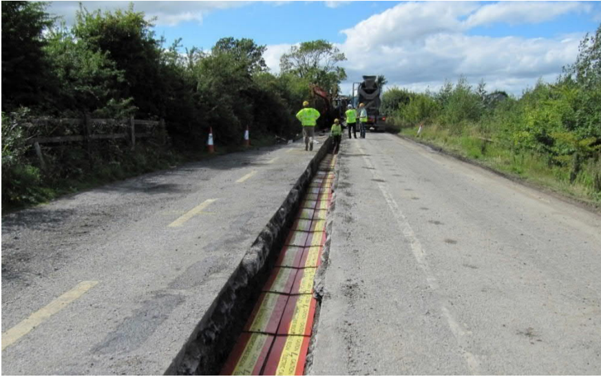
Figure 11: HVDC Cable Trench in Road
