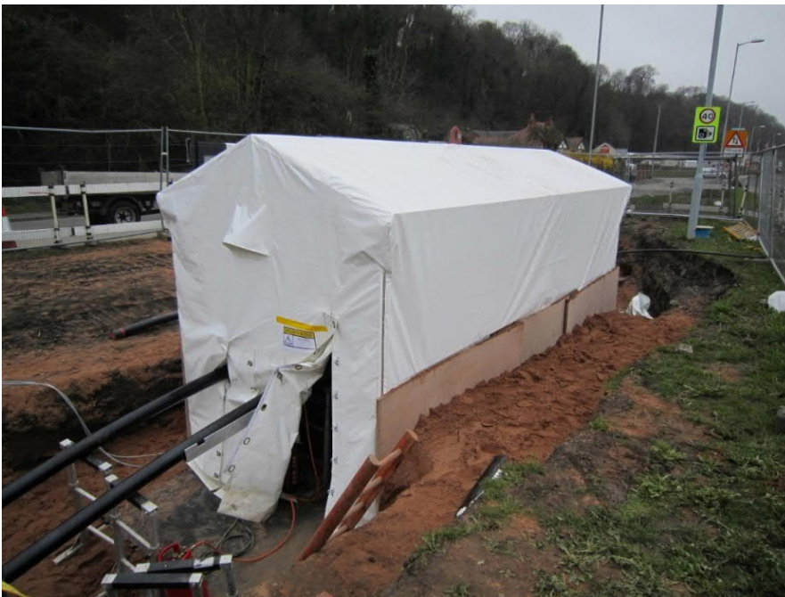
Figure 12: HVDC Cable Jointing Bay Shelter
