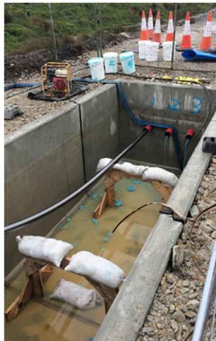
Figure 17: HVAC joint chamber with one cable pulled in preparation for jointing
