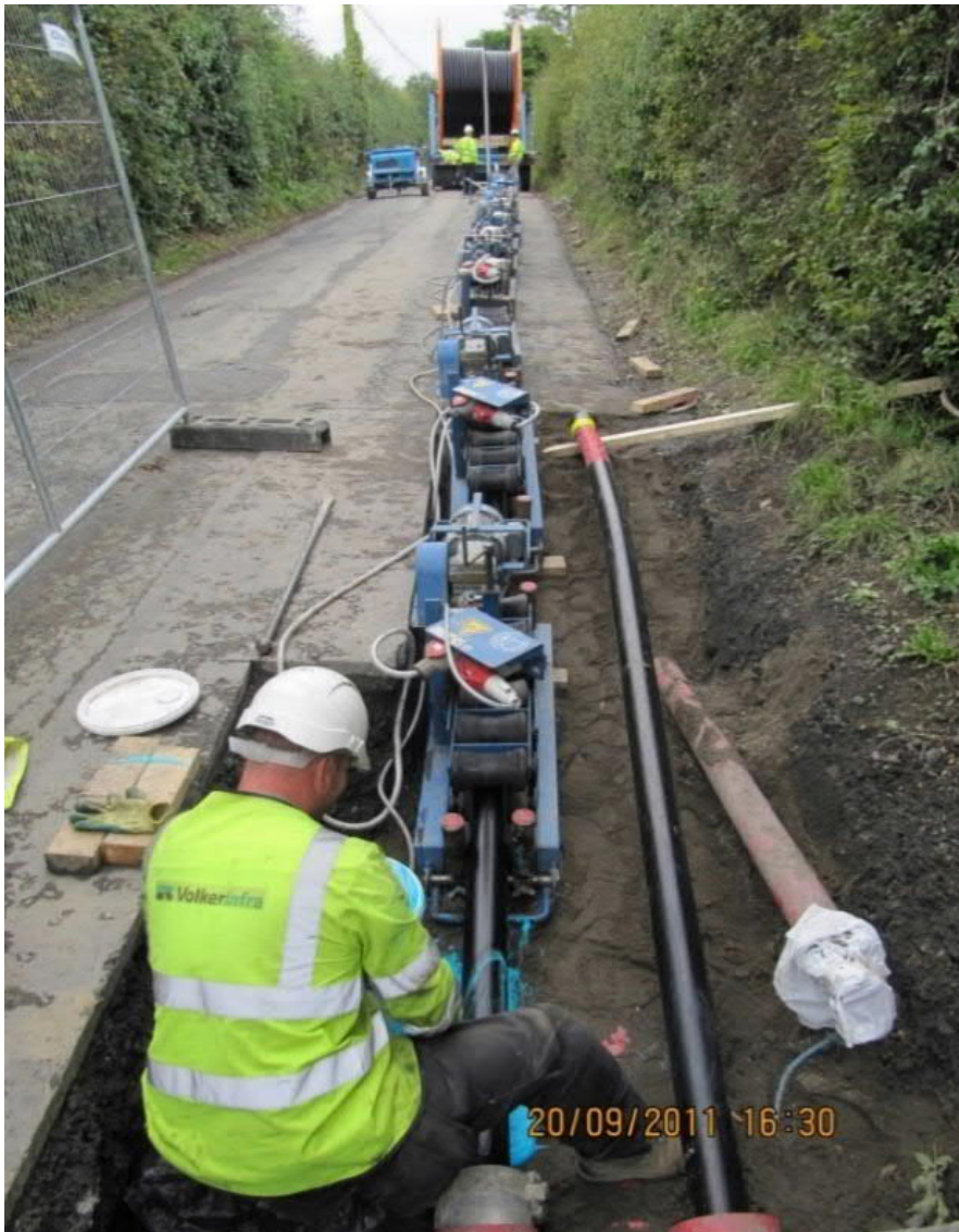
Figure 13: HVDC Cable Laying
