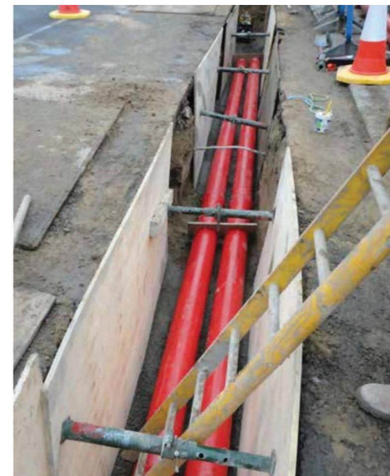
Figure 6 Installation of plastic ducts
