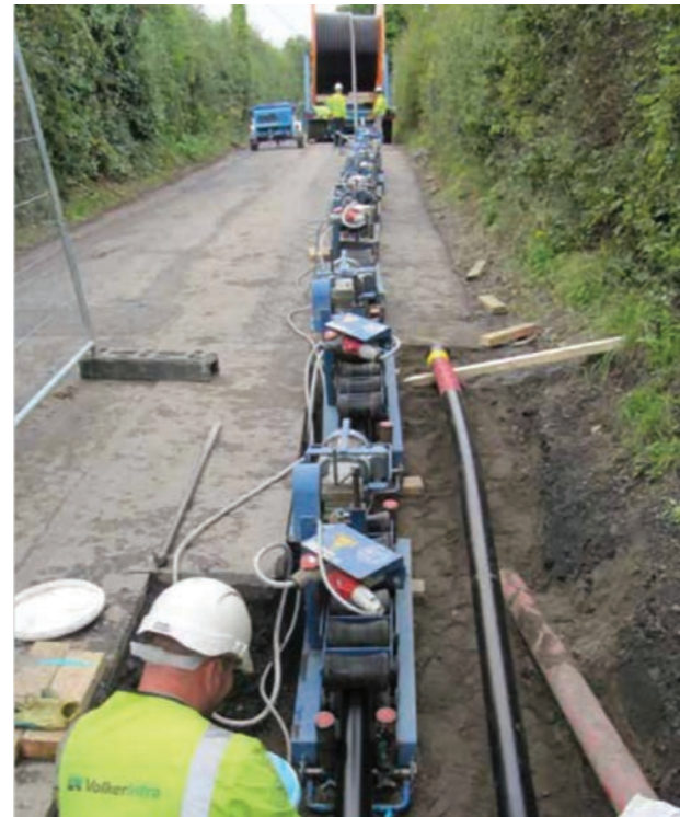
Figure 8 Installation of cable into the ducts
