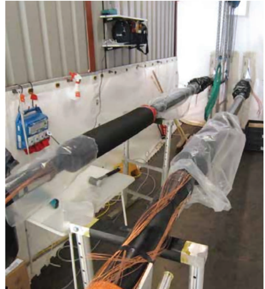
Figure 9 Jointing of cable sections
