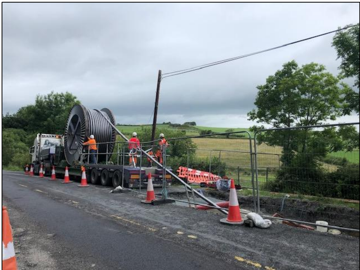
Figure 3.5: Photograph of cable installation into the pre-laid ducts at a joint bay (Source: EirGrid)
