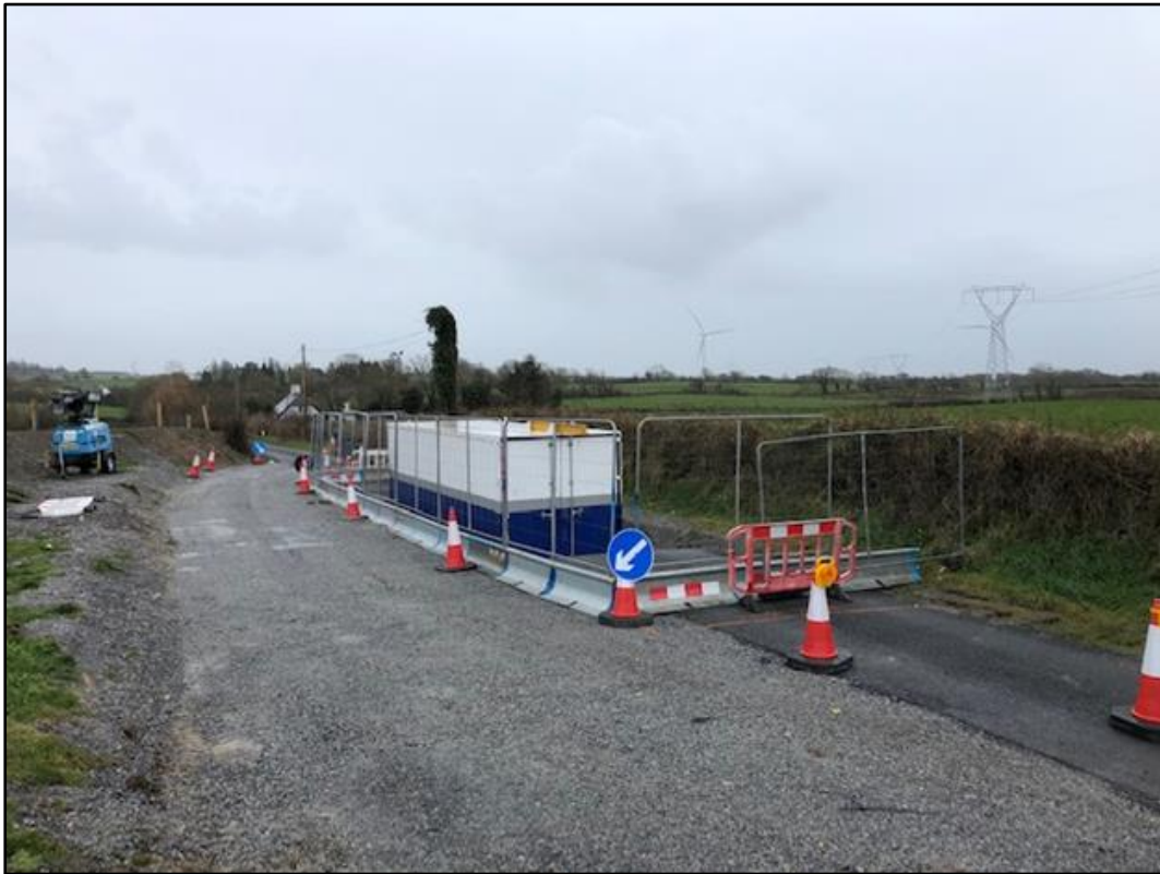
Figure 3.6: Typical HVDC Cable Jointing Bay enclosure (Source: EirGrid)
