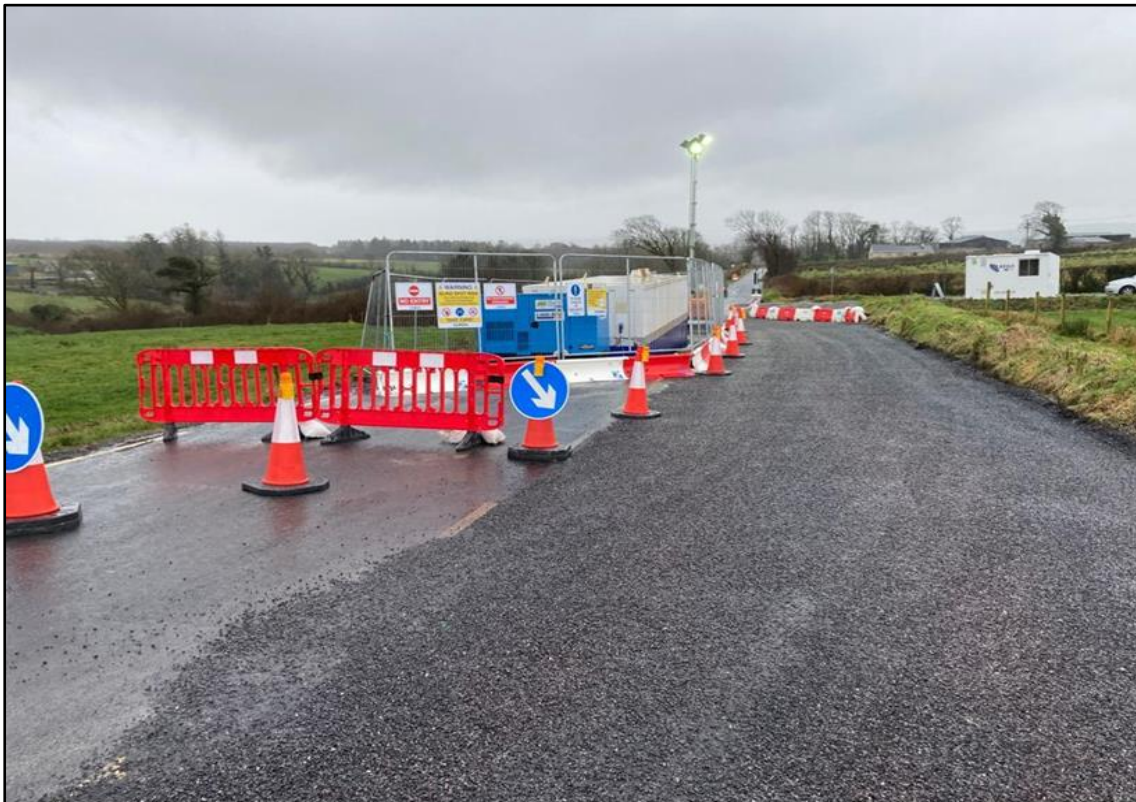
Figure 3.4: Photograph of Passing Bay in operation. The steel structure in the middle of the picture behind the Harris fence has been placed on top of the joint bay to form an enclosed workspace where cable jointing is taking place. (Source: EirGrid)
