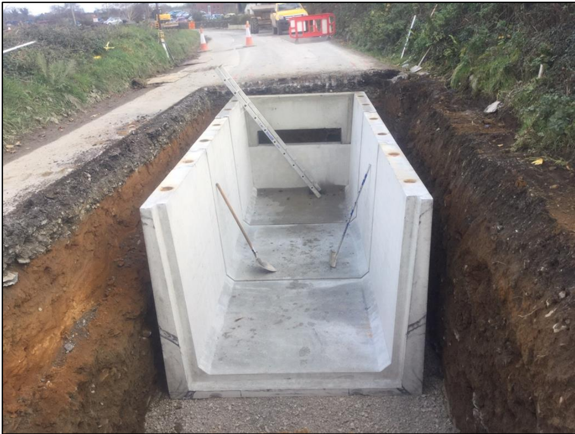
Figure 3.2: Typical Joint Bay under construction.
