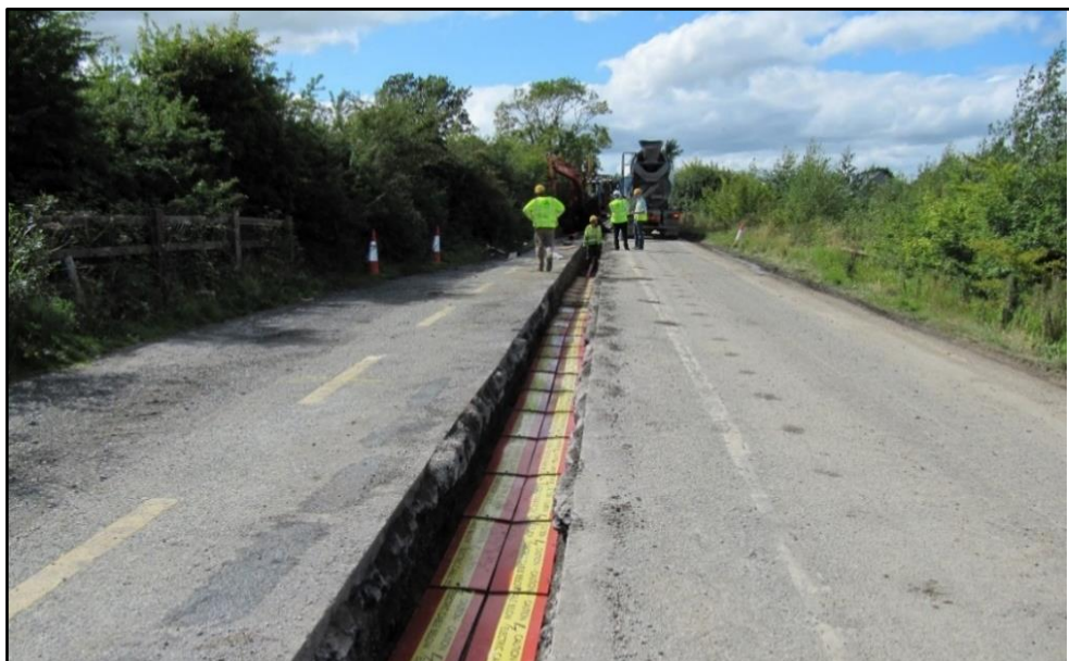
Figure 3.1: Typical DC trench laid in the public road (source EirGrid)
