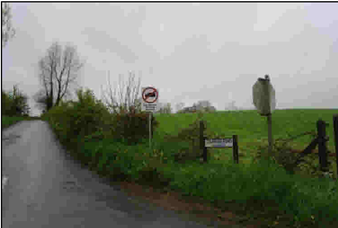
Illustration 18.3 - Weight Restriction Advisory Sign (Culverog Road)
