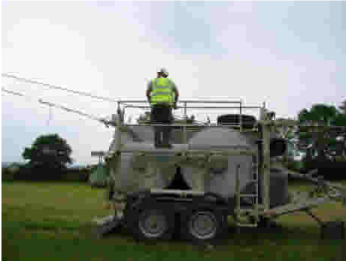
Illustration 5.8: Winching machine for stringing operation.
