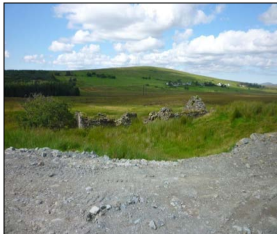
Example of a crushed stone access road installed to avoid undesignated farmstead in ruin
