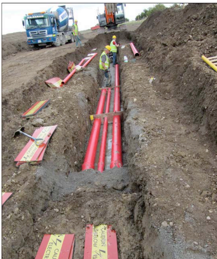
Underground cable construction on agricultural land
