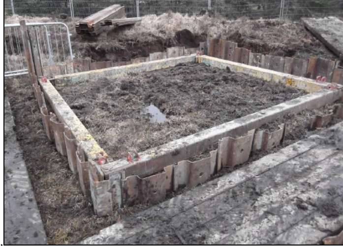
Donegal 110kV Project Sheet Piling used in poor ground for angle mast foundation pit courtesy of Byrne Mullins & Associates
