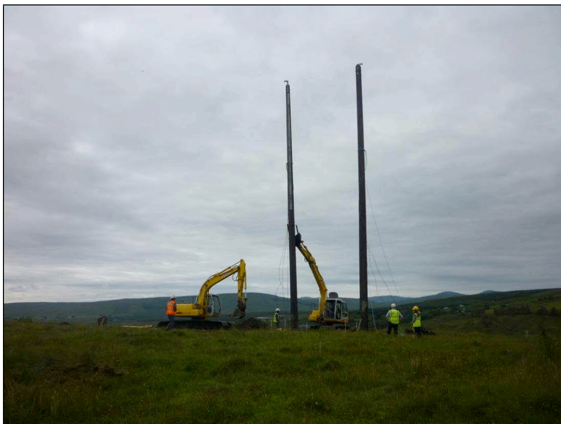
Construction of wooden pole set support structure for Donegal 110 kV Project (Binbane – Letterkenny)
