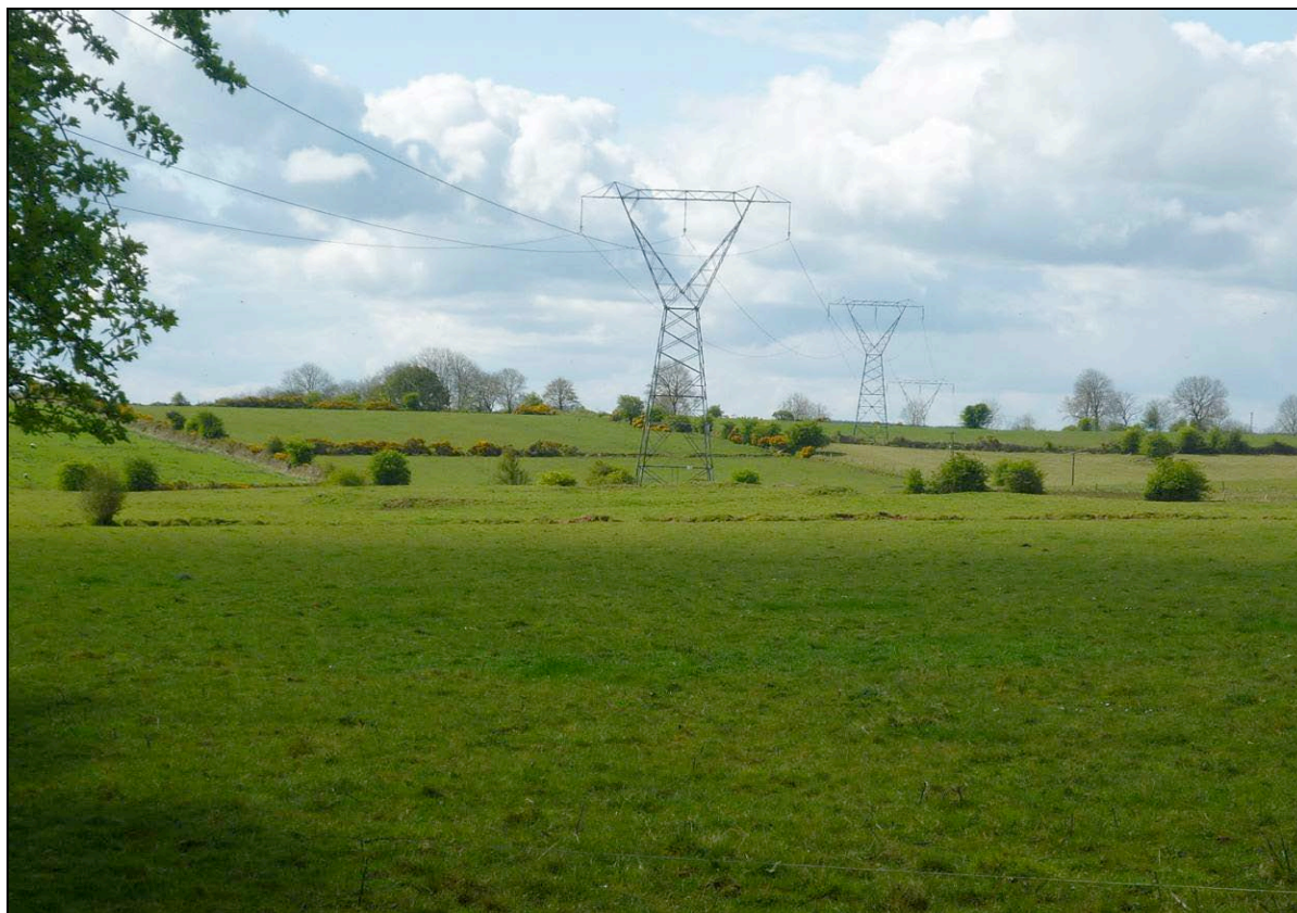
Example of a typical 220 kV intermediate tower design along the Cashla – Flagford overhead line showing a ringfort (RO022-054064), Co Roscommon
