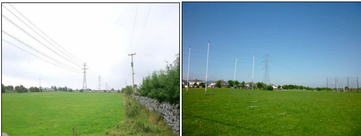
Typical 110 kV double circuit structure in close proximity to an amenity area
