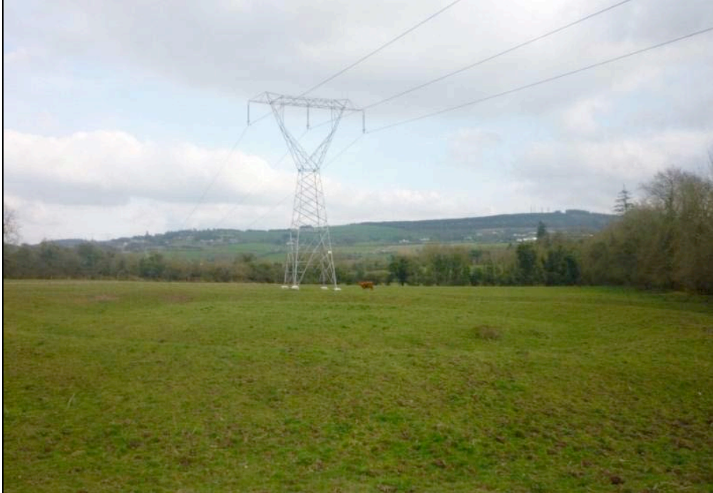
This 220kV intermediate tower is located on the outer bank of a ring barrow (DU021-039). It has a significant direct impact on the monument and setting. (Carrickmines – Maynooth 220 kV, Co. Dublin)
