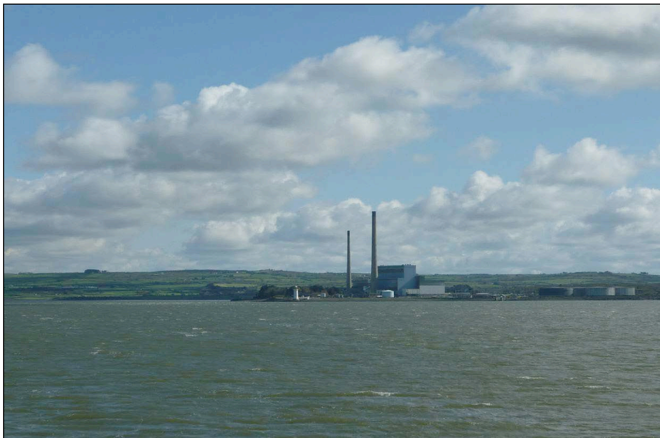
View to Tarbert Power Station, Co Kerry recorded as a Battery (KE003-002--) and a Bastioned Fort (KE003-001--) in the Record of Monuments and Places (RMP)
