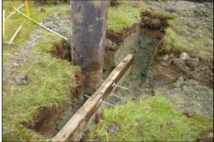
Trench for pole and sleepers used to stabilise pole
