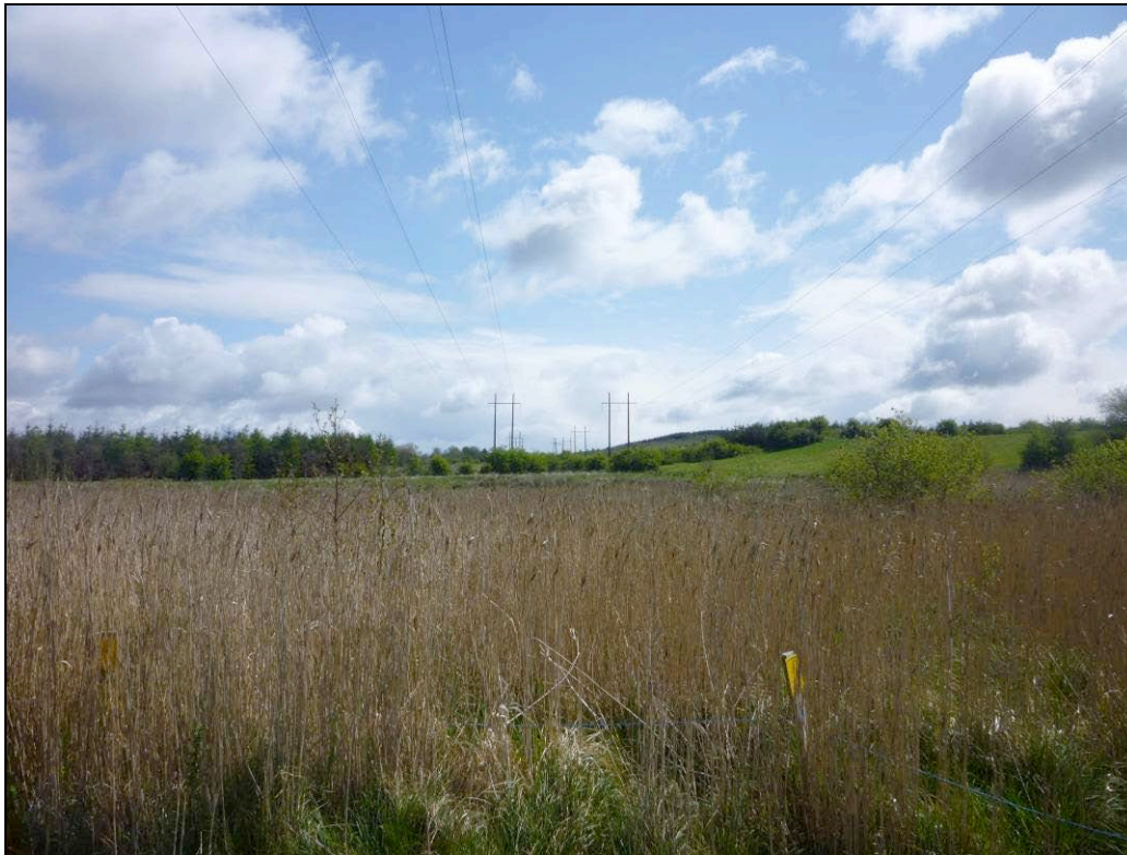
Example of a typical 110kV support structure in the form of double wood polesets (Co Sligo)
