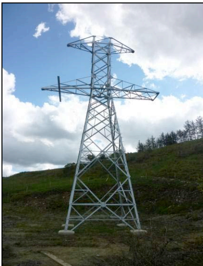
Typical Angle Tower (110 kV) and structure foundation designed in response to a wetland environment
