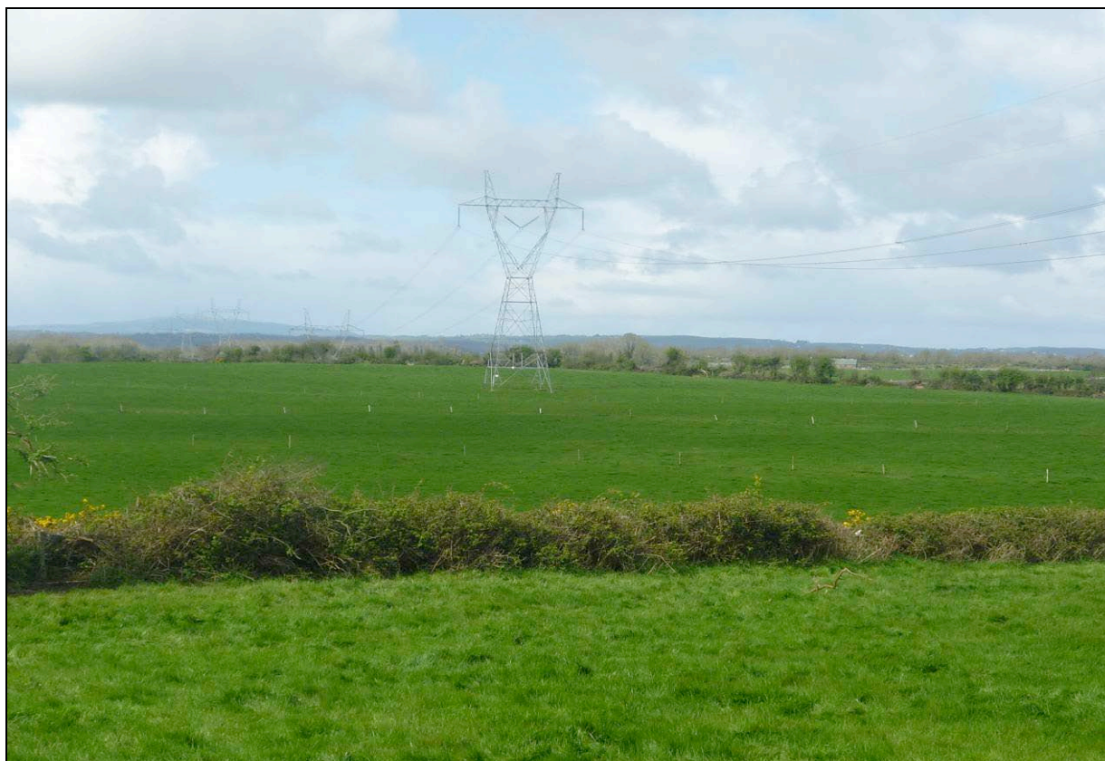
Example of a typical 400 kV intermediate tower design along the Dunstown-Moneypoint overhead line with a view towards a low visibility ceremonial enclosure (CL042-020), Co Clare
