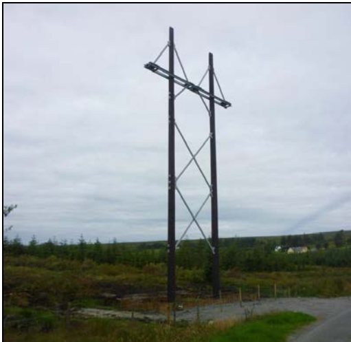
Typical 110 kV steel braced poleset
