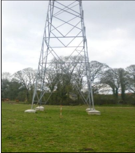
Typical foundation footings Carrickmines – Maynooth 220 kV, Co. Dublin
