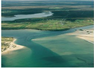
Corrib Gas Pipeline (post Rosport 5)
