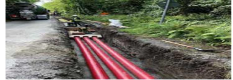
A typical cable duct installation in the road
