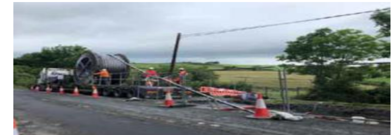
Cables being pulled into the ducts and jointing bay
