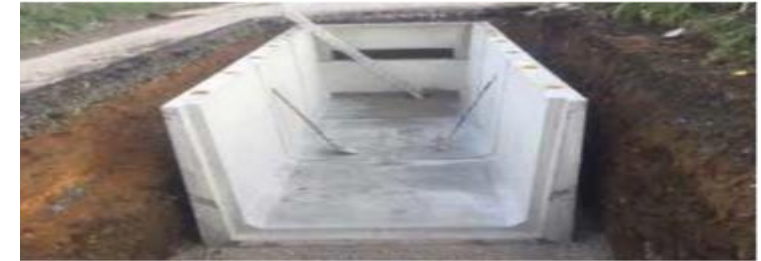
A typical jointing bay where cables are connected
