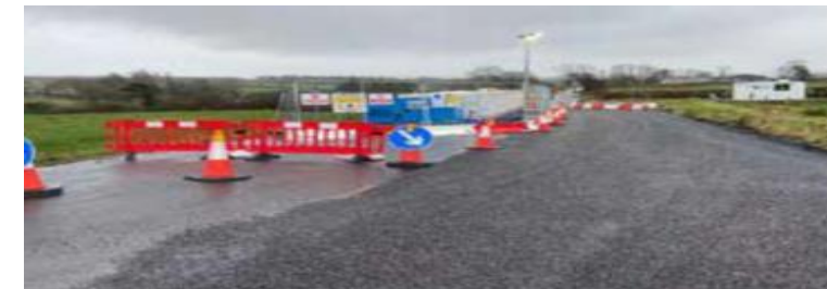
A typical passing bay in operation during cable jointing
