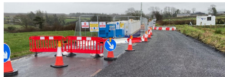
Figure 7: A typical passing bay in operation during cable jointing
