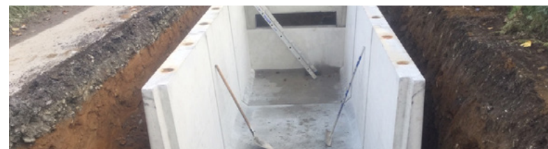
Figure 5: A typical jointing bay where cables are connected
