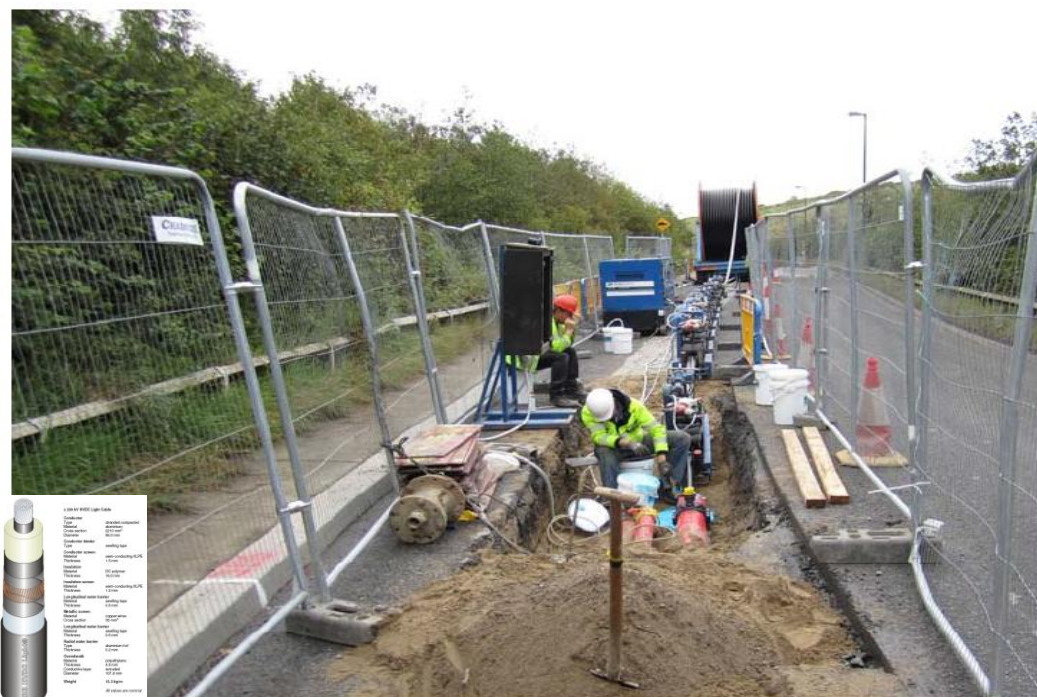
Above: A drum containing 500m of land cable is off-loaded and guided along cable rollers and pulled through the pre-installed cable ducts. The entire interconnector cable took almost 2 years to manufacture.
