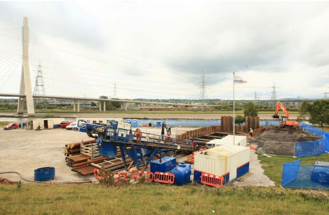
Above: A 250 tonne Horizontal Directional Drill bores a 600m crossing below the River Dee in Wales.
