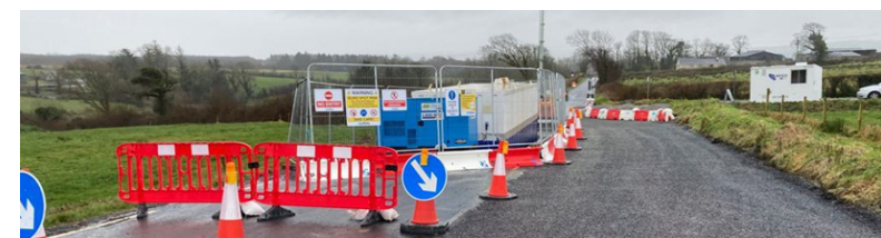
Figure 7: A typical passing bay in operation during cable jointing
