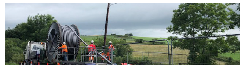
Figure 6: Cables being pulled into the ducts and jointing bay
