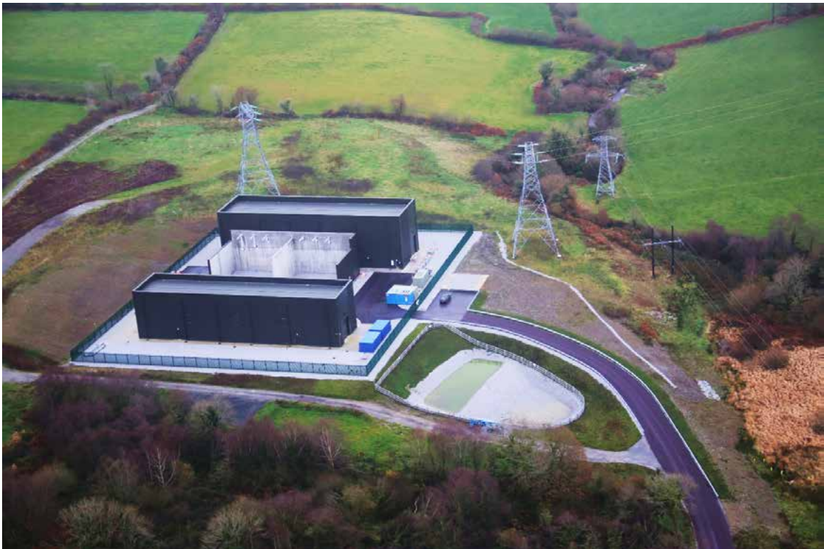
Figure 3.13: 220 kV Gas-insulated substation
