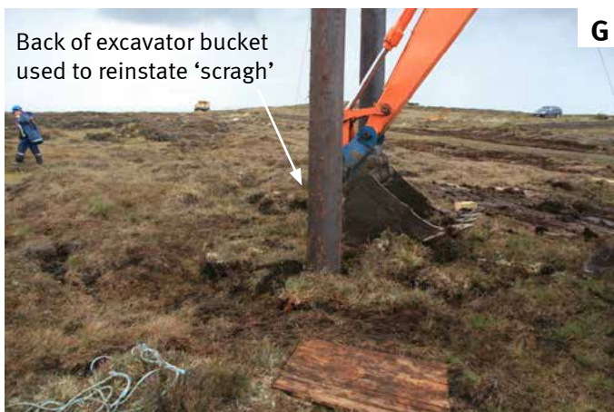
Figure 5.5: Habitat protection measures implemented during poleset construction
