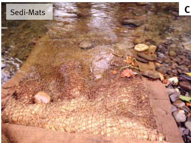
Figure 5.5: Silt Fencing (a & b), Sedi-Mats (c) and Silt Curtains (d)
