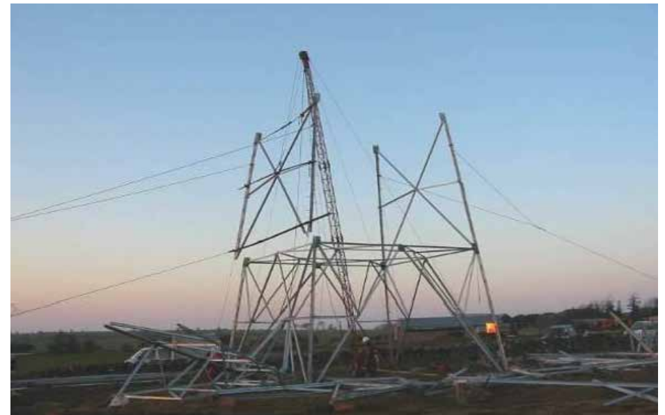
Figure 3.6: Erection of Tower
