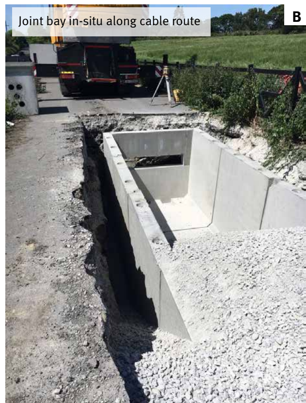
Figure 3.10: Cable duct and joint bay installation
