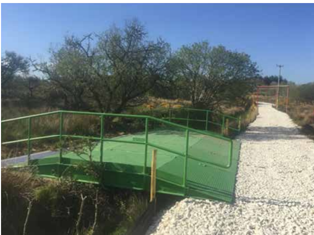
Figure 5.7: Examples of clear-span structures over watercourses
