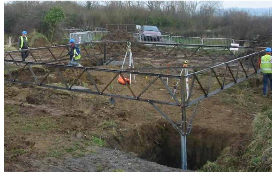
Figure 3.5b: Tower foundation during construction
