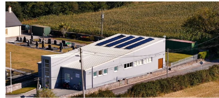
Solar panels on the Ballintotis Community Centre.
