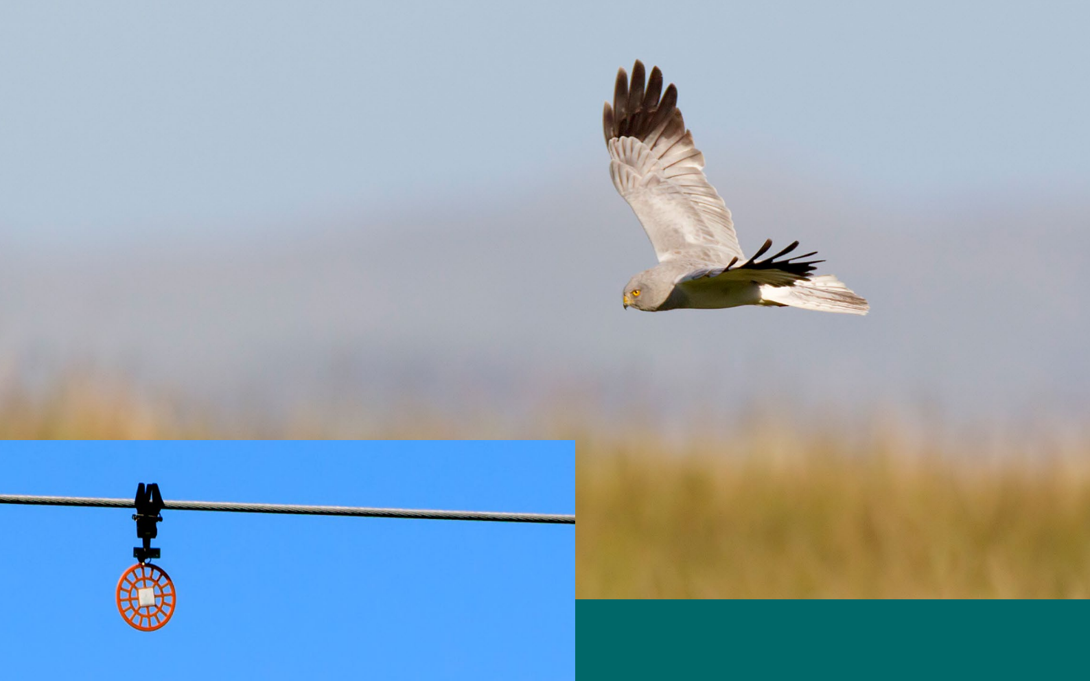
An example of a bird flight diverter installed on an electricity cable.
