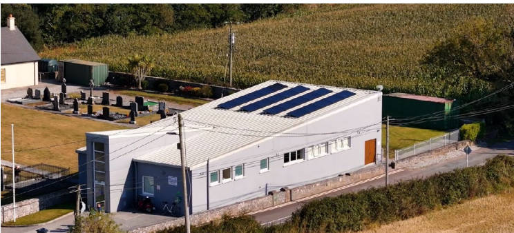
Solar panels on the Ballintotis Community Centre.
