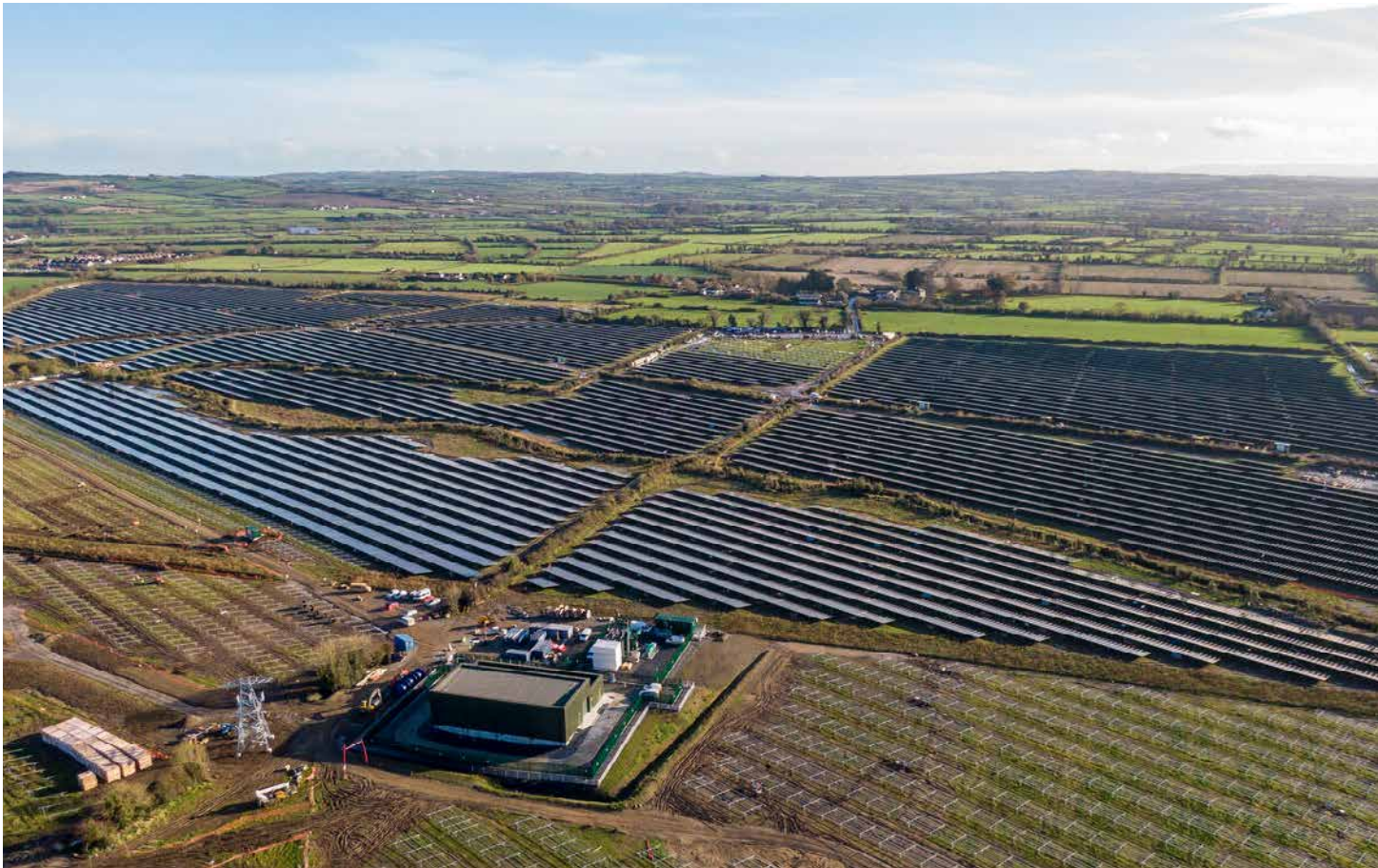
Rathnaskilloge 110 kV Station, Co Waterford. This is a RESS 2 project that was connected in March 2025.
