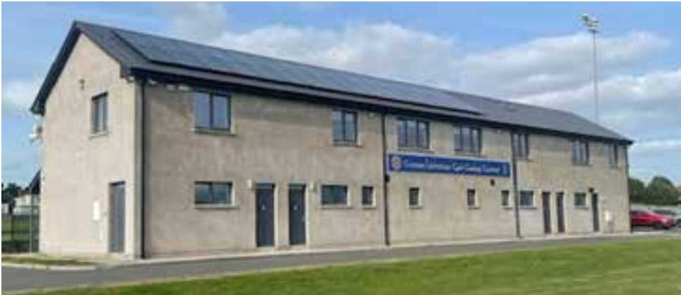
Solar panels at Carrigtwohill GAA Club, Co. Cork.
