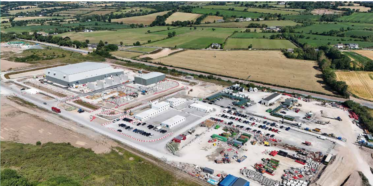
Aerial view of Ballyadam converter station
