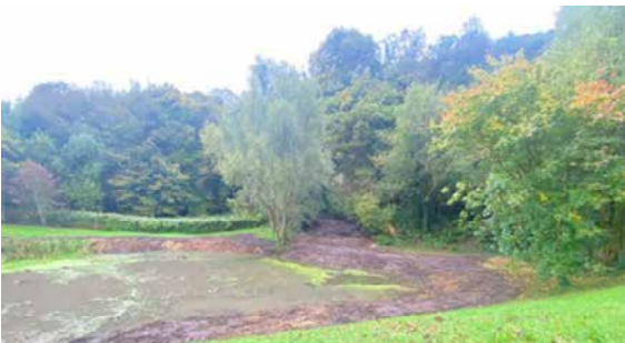
The Keane Park Pond restoration project Youghal Blue and Green Community Network, Co Cork.
