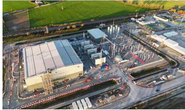
Construction progress at the Celtic Interconnector Converter Station at Ballyadam, Co. Cork.
