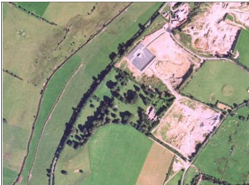
Illus. C 91 Aerial photograph showing the mature woodland estate of Castleruddery House, the enclosure site (WI021-026).
