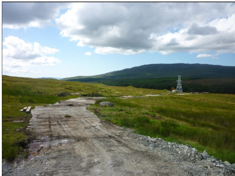
Illus. C 9 Temporary bog mat access route to tower (No 180)
