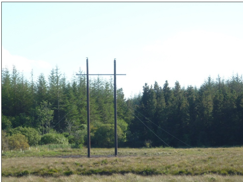
Stay lines in place, Donegal 110 kV Project
