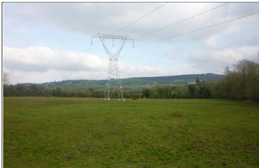
Illus. C 99 Barrow (DU021-039), taken from the north looking south
