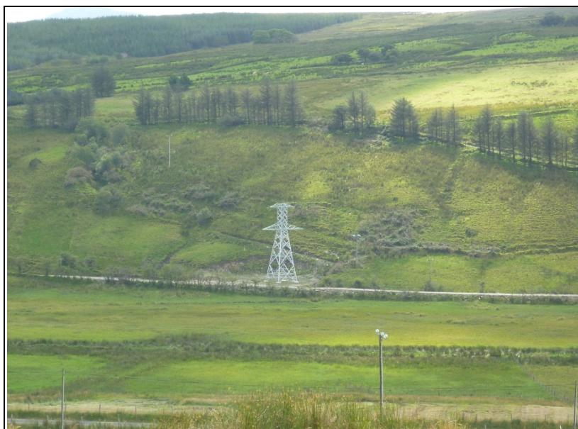
Illus. C 7 Tower (No 215) adjacent to dismantled railway embankment
