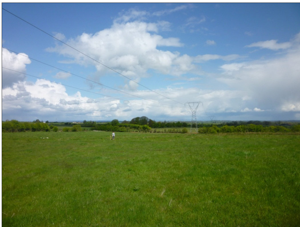
Illus. C 53 Transmission line and towers over road/trackway (RO022-057061)
