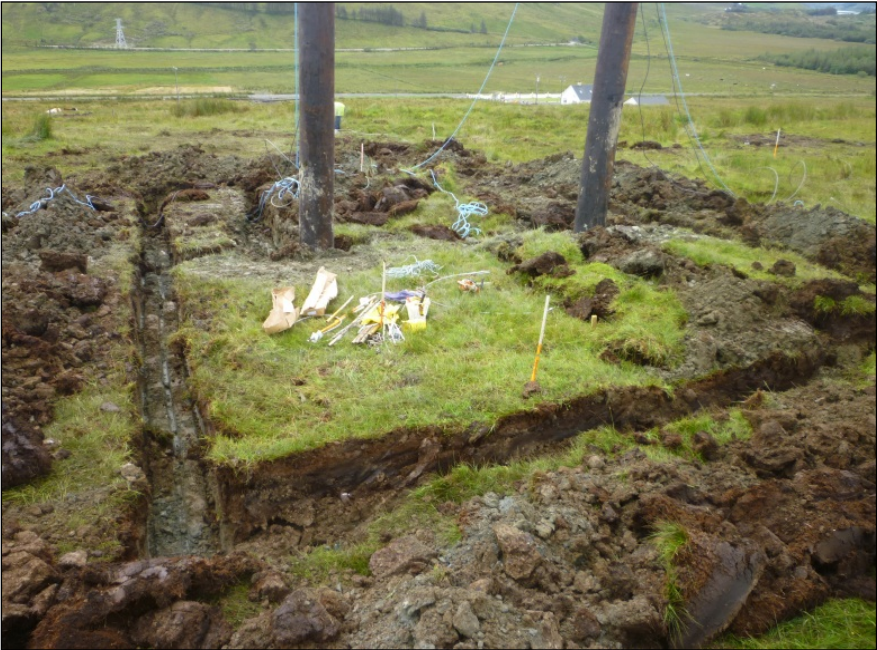
Earth ring on Donegal 110kV Project
