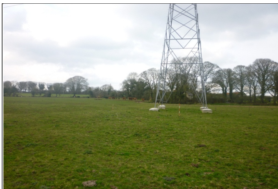
Illus. C 100 Transmission tower located on the outer southern bank of the barrow site, taken from the south west
