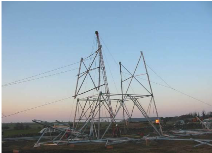
Installation of tower using a derrick pole at the base
