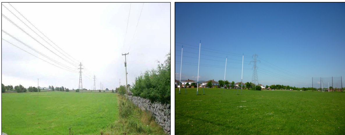
Typical 110 kV double circuit structures
