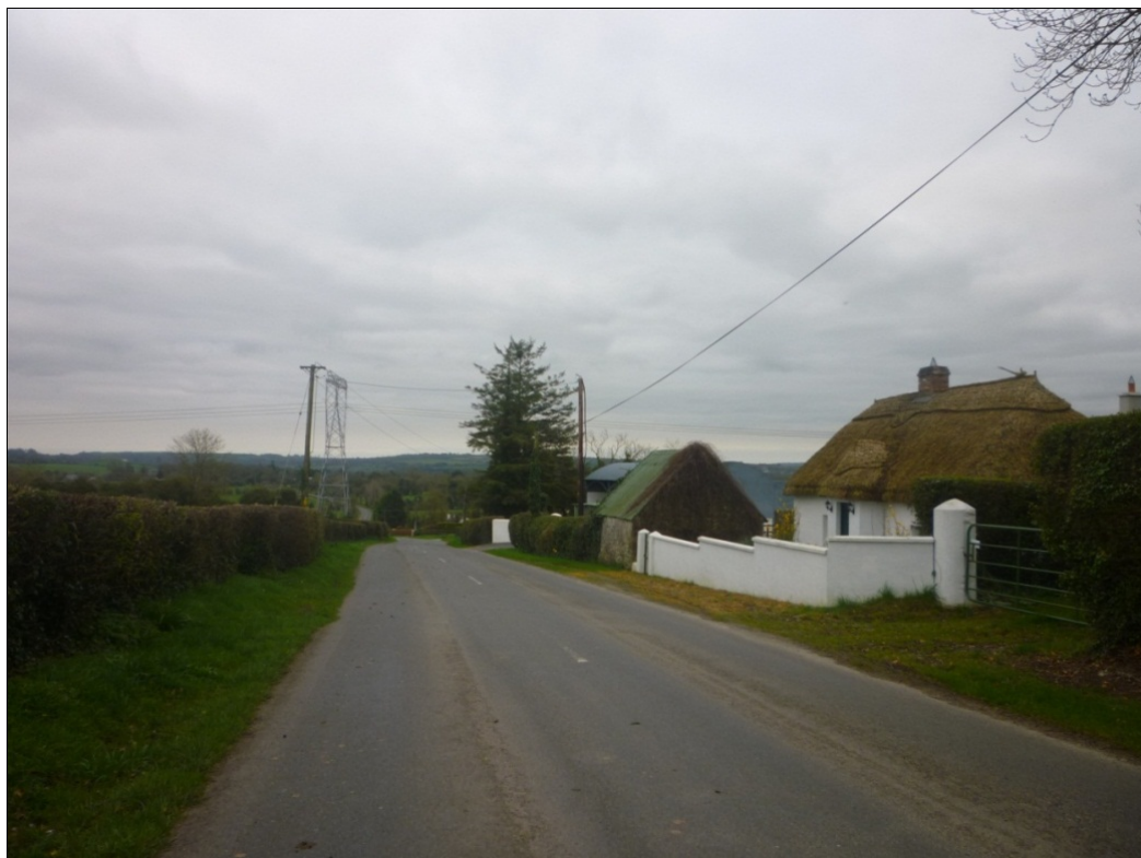
Illus. C 83 A thatched roadside vernacular cottage is located approx. 92m west and uphill of the steel tower.
