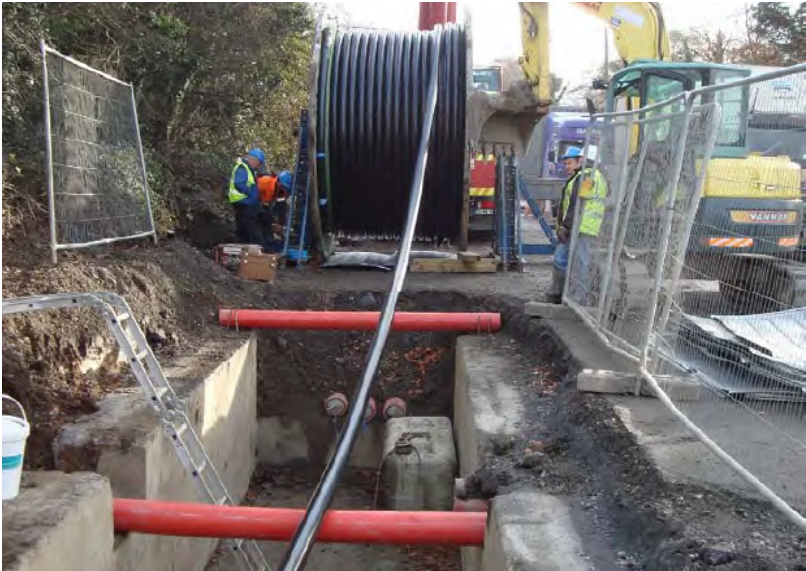
Typical HV Cable Installation
