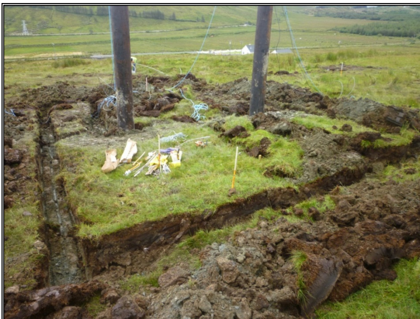
Illus. C 4 Excavation trench required for the earth ring
