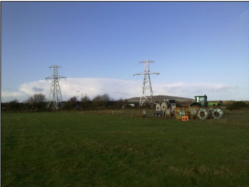
Conductor stringing equipment
