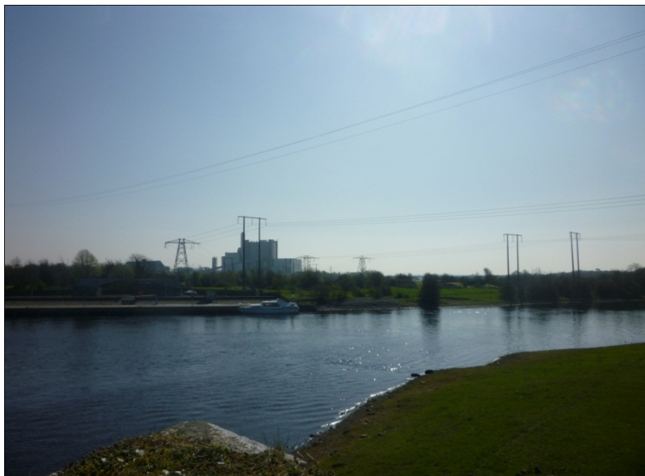
Illus. C 48 Views from the bridge and the bastioned fort
