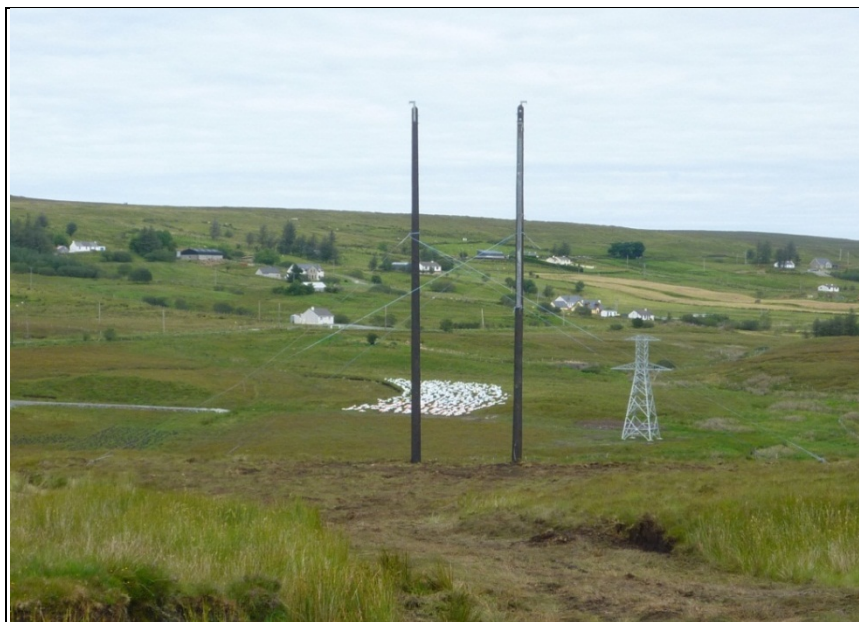
Illus. C 5 Finished poleset (No 219) with stay lines in place
