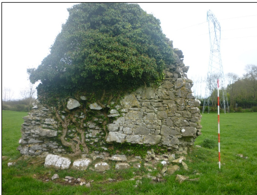
Illus. C 35 View east towards the surviving castle wall and the steel lattice tower to the southeast
