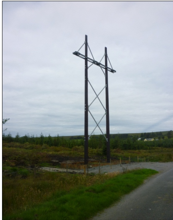
Braced double wood poleset
