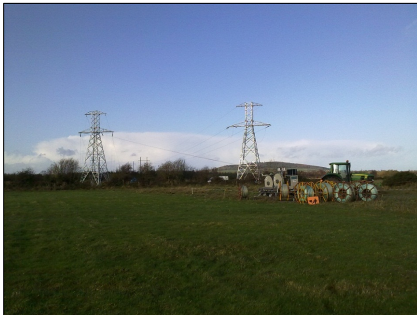
Conductor stringing equipment
