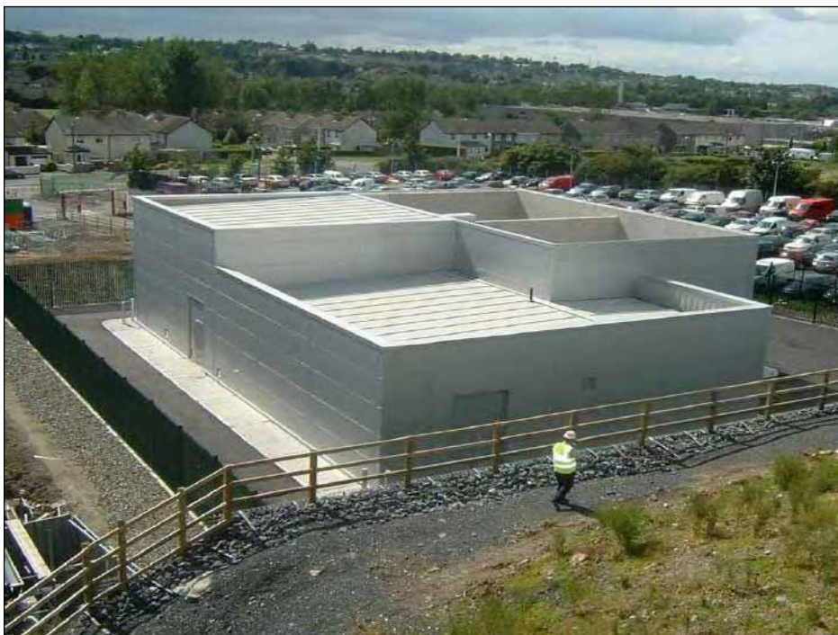
Example of a typical indoor GIS substation, Co Limerick
