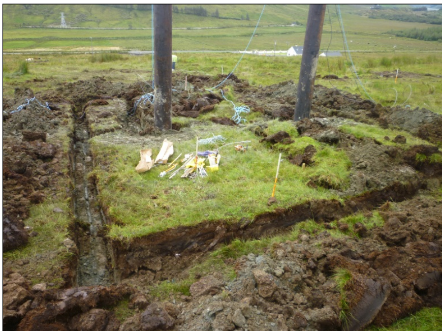
Earth ring on Donegal 110kV Project
