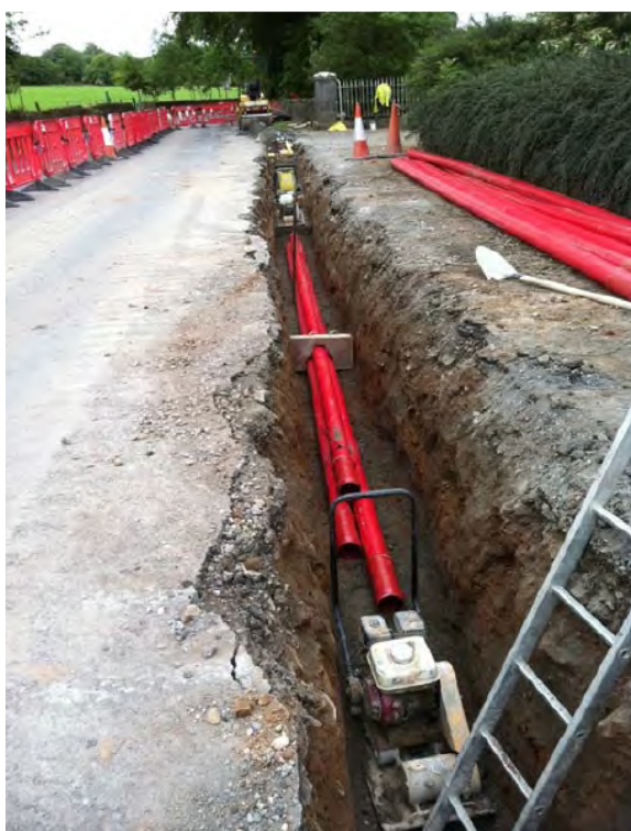
Typical 110kV Trench Excavation (Ducts in Trefoil Formation)
