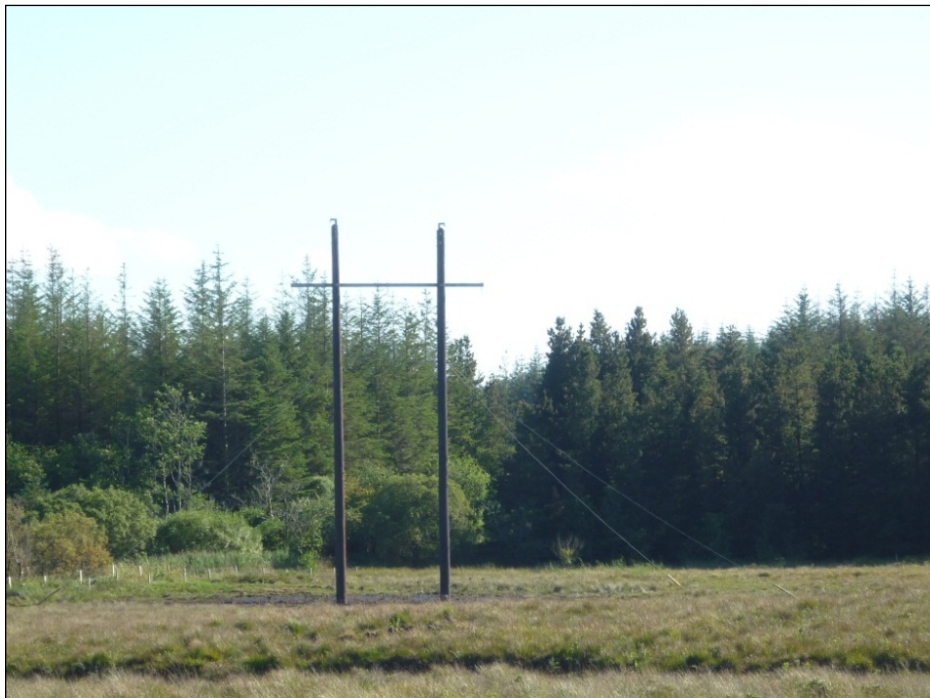
Stay lines in place, Donegal 110 kV Project
