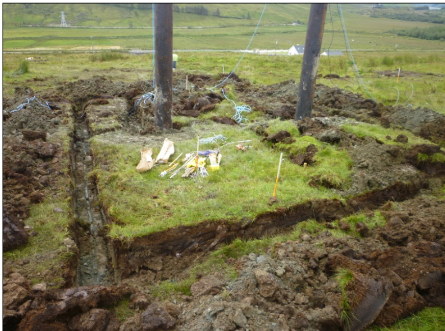
Earth ring on Donegal 110kV Project
