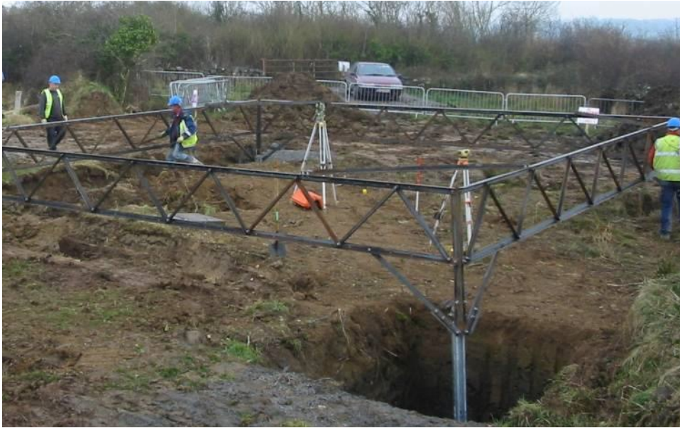
Figure 3.9: 400kV tower foundations being prepared for concreting (ESBI 2012c)
