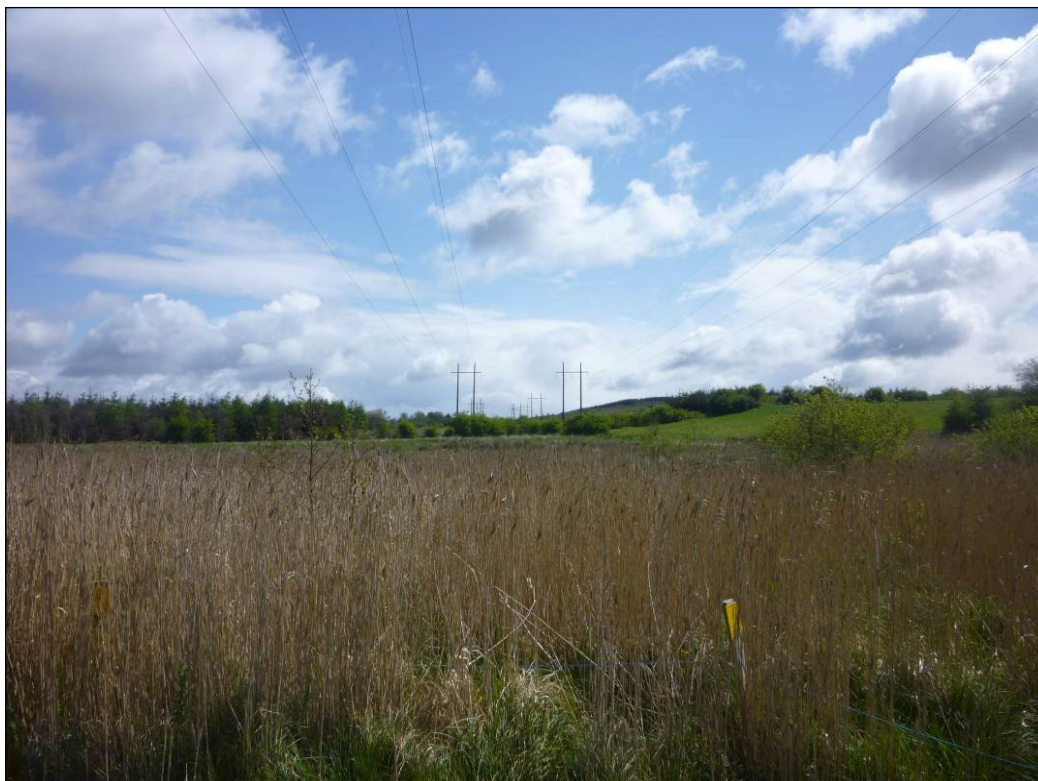
Example of a typical 110kV single-circuit double wood polesets with earthwire (Co Sligo)
