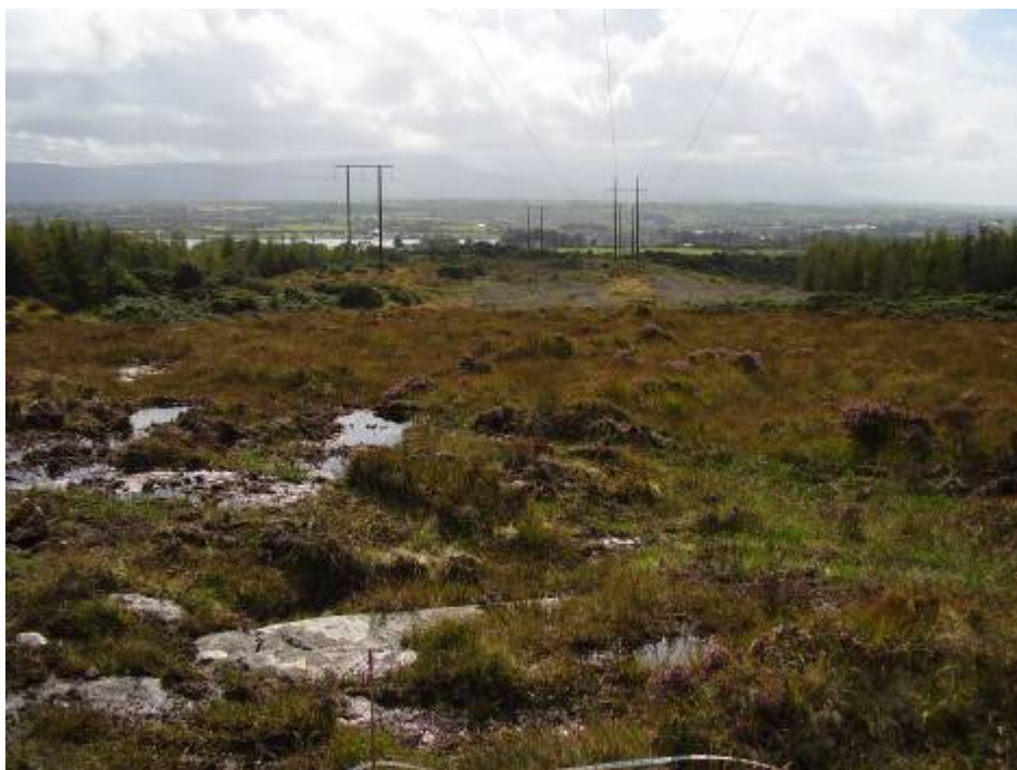
Figure 3.2: Example of a 110kV transmission line showing wooden polesets
