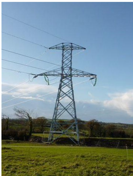
Figure 3.5: Typical 110kV angle tower in situ (ESBI 2012c).
