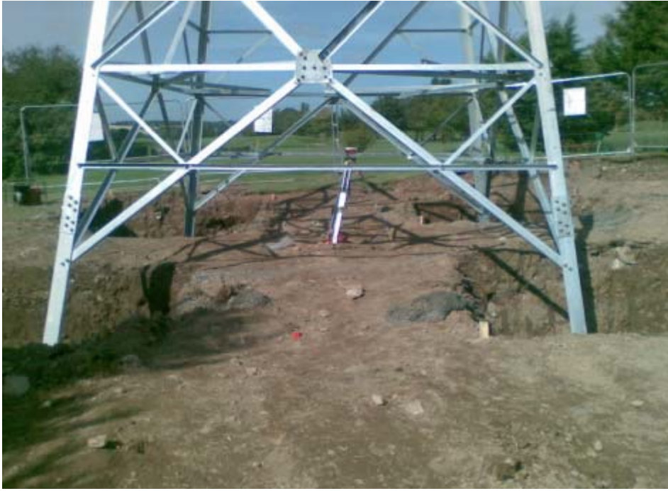
Figure 3.7: Photograph of typical tower base with excavations (ESBI 2012b).
