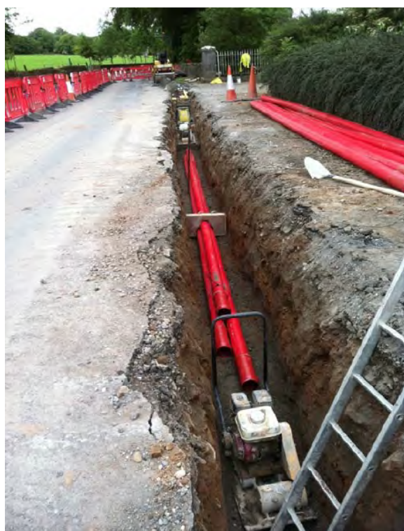
Typical 110kV Trench Excavation (Ducts in Trefoil Formation)
