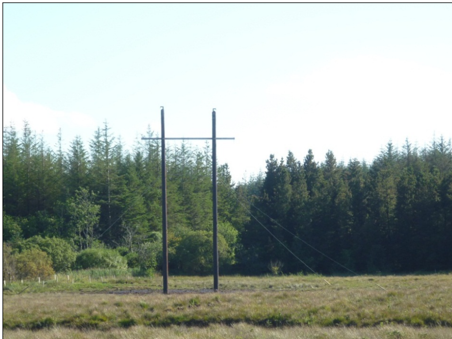
Stay lines in place, Donegal 110 kV Project
