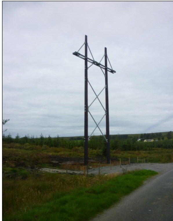
Braced double wood poleset
