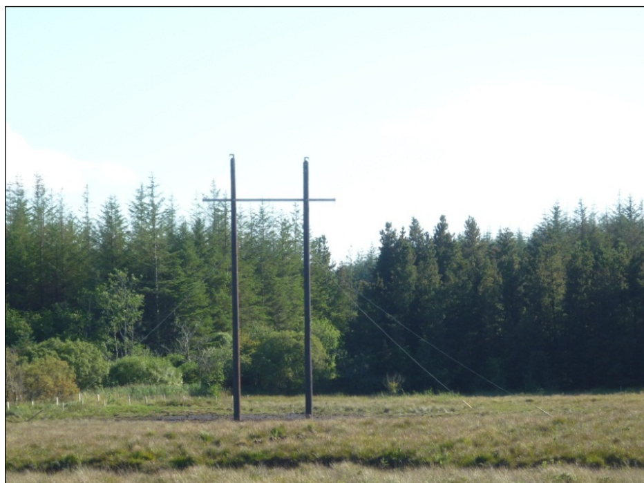
Stay lines in place, Donegal 110 kV Project
