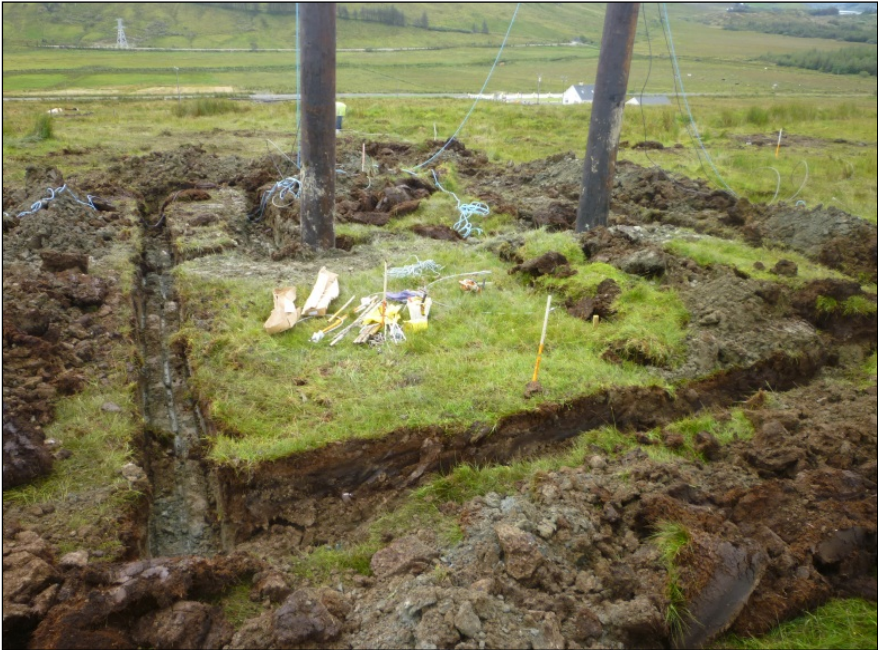
Earth ring on Donegal 110kV Project
