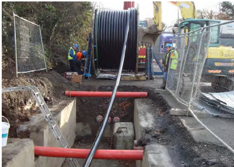
Typical HV Cable Installation
