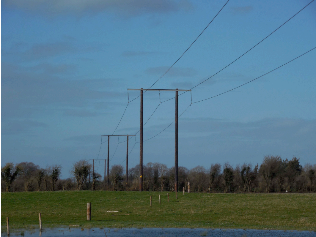
Figure 16: Study site at Clonony More (Shannonbridge-Thurles 110kV line)
