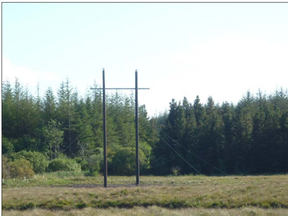
Stay lines in place, Donegal 110 kV Project
