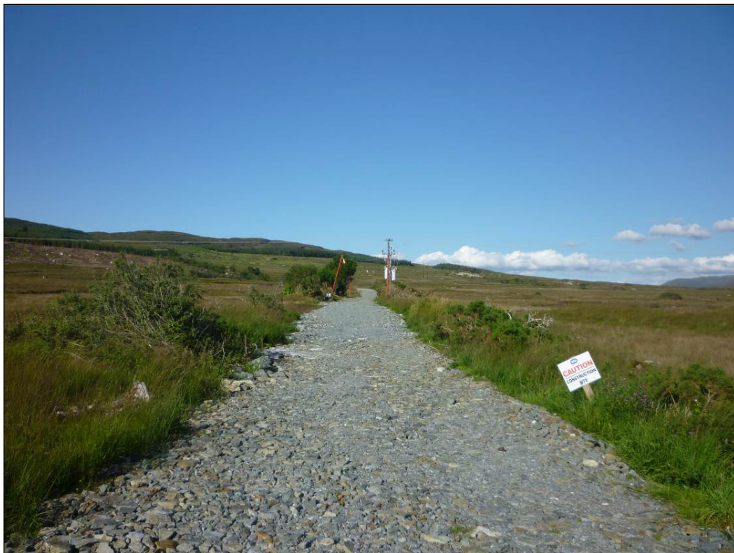
Example of a newly built access route for a transmission project, Co. Donegal
