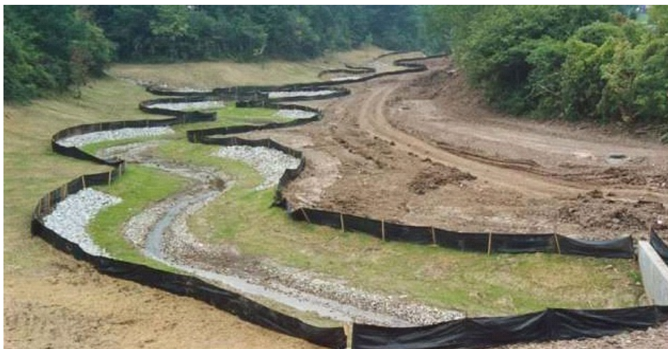
Figure 2.4 Example of a silt fence preventing sediment release into ditch/channel
