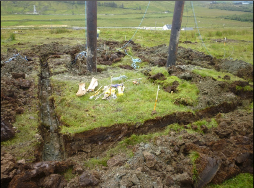
Earth ring on Donegal 110kV Project
