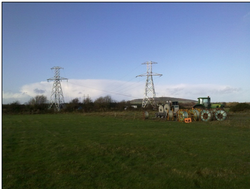
Conductor stringing equipment
