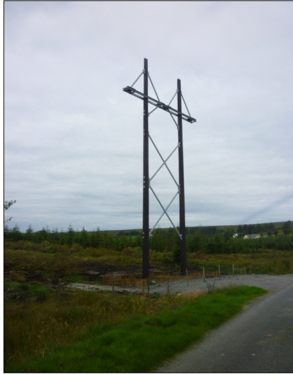
Braced double wood poleset
