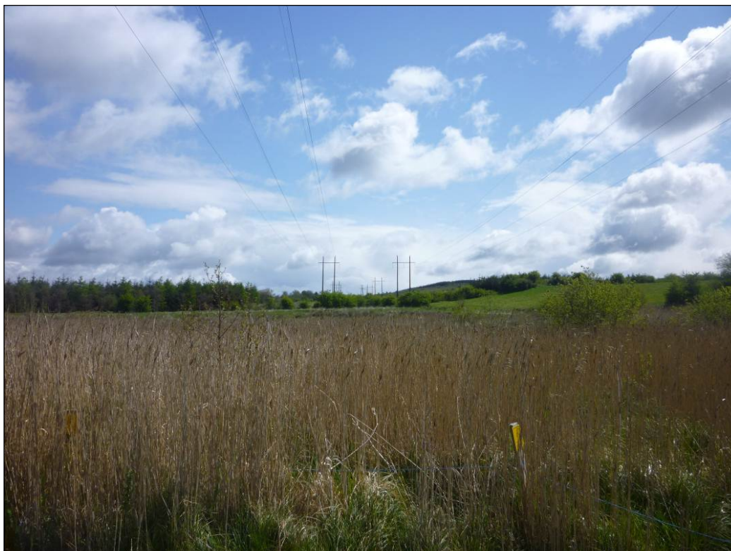
Example of a typical 110kV single-circuit double wood polesets with earthwire (Co Sligo)
