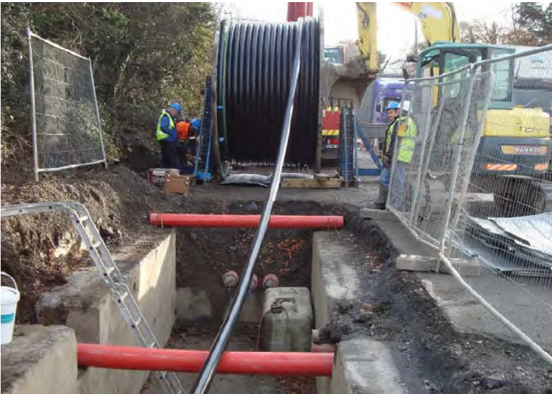
Typical HV Cable Installation
