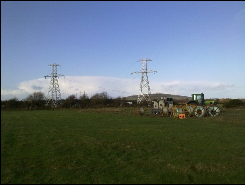
Conductor stringing equipment
