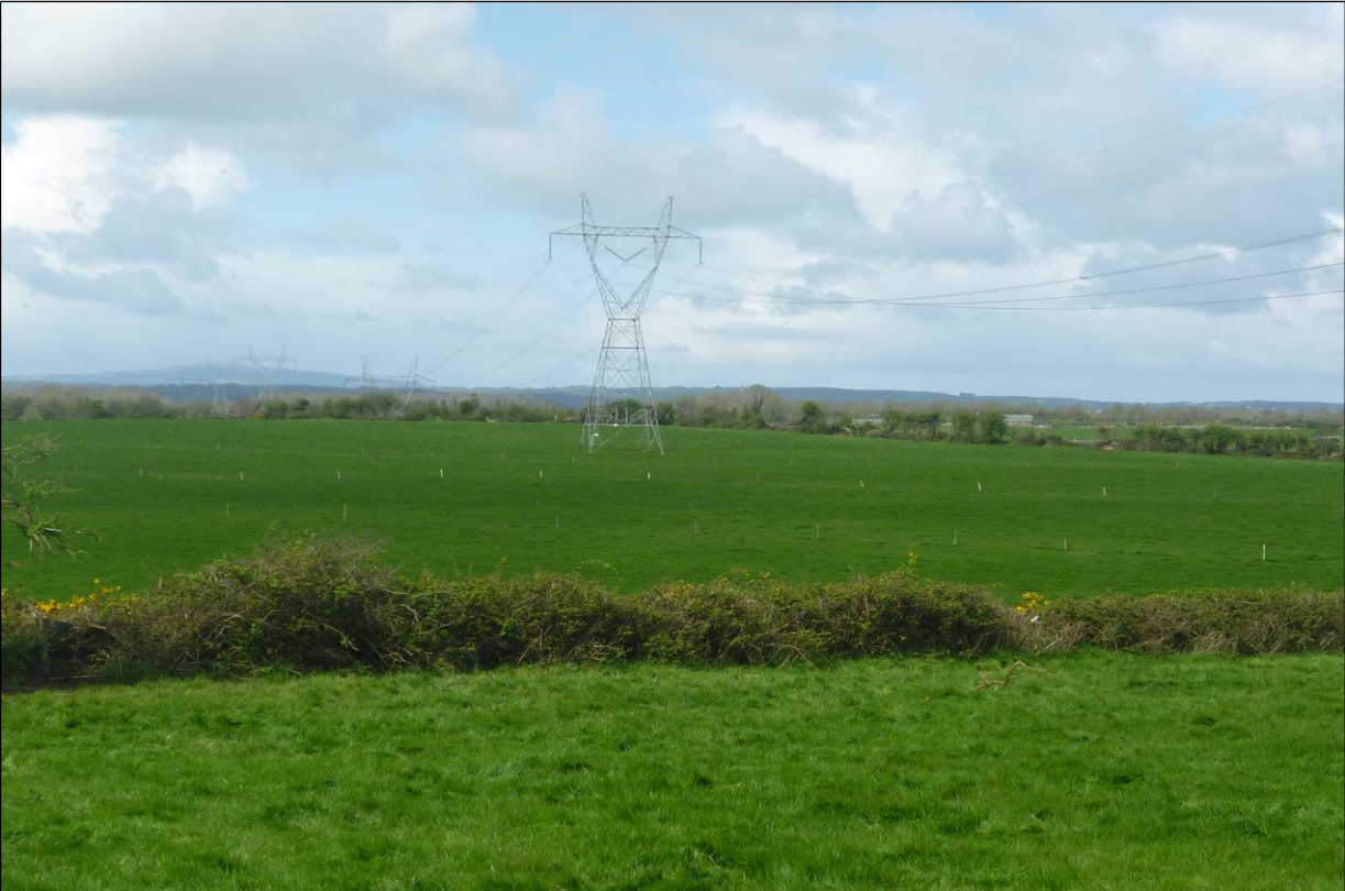
Example of a 400 kV intermediate tower design along the Dunstown-Moneypoint overhead line, Co Clare
