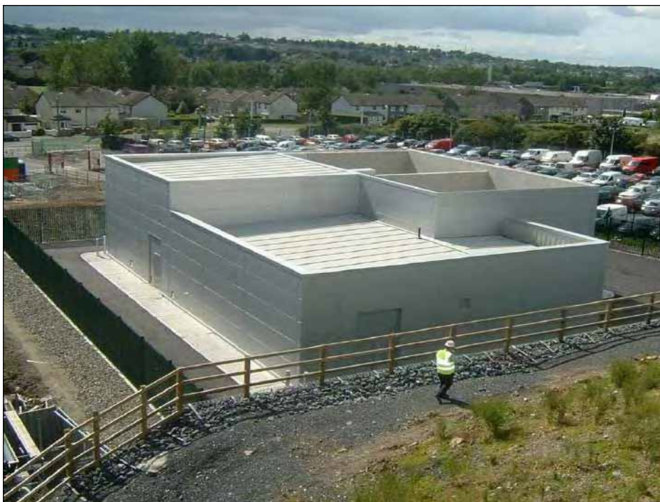
Example of a typical indoor GIS substation, Co Limerick
