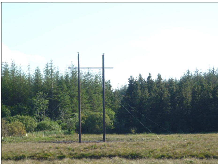
Stay lines in place, Donegal 110 kV Project
