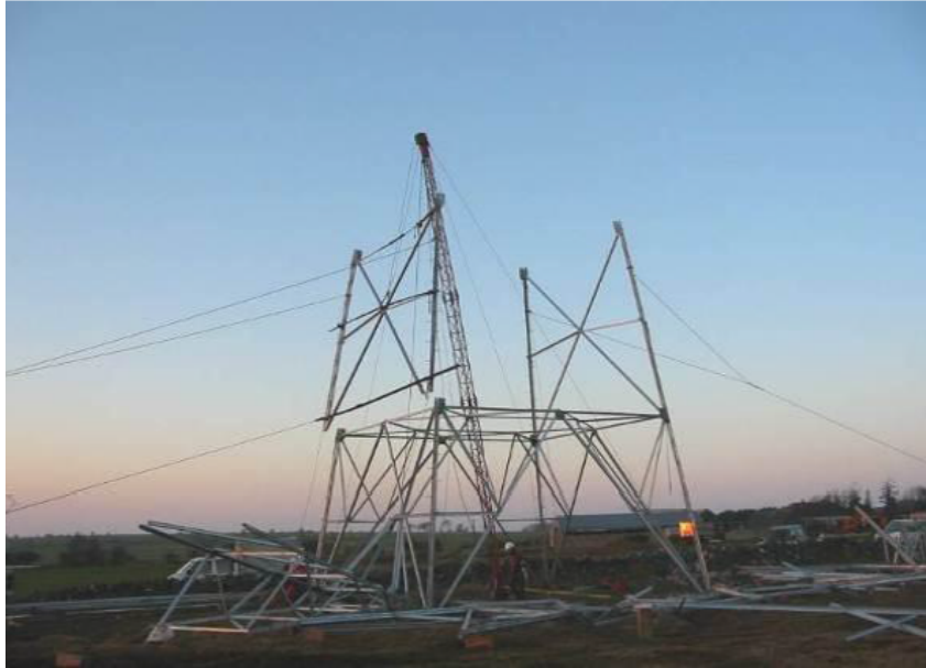
Installation of tower using a derrick pole at the base
