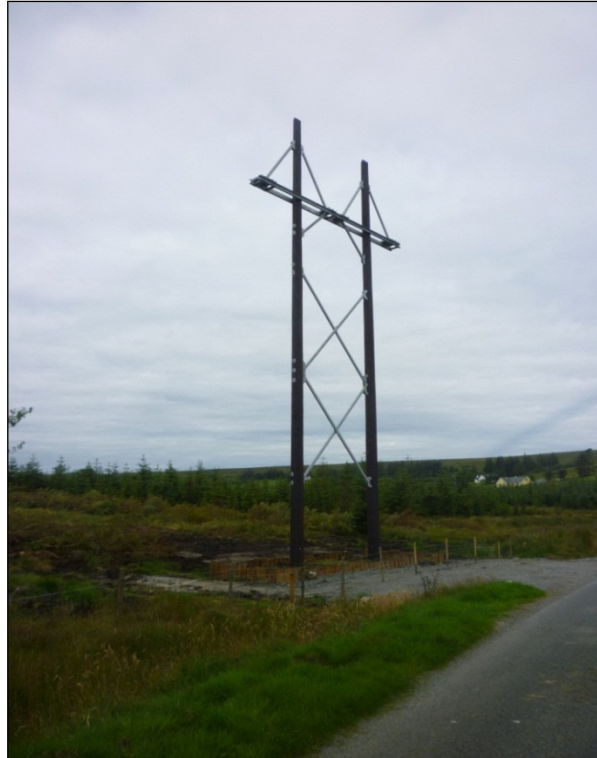
Braced double wood poleset
