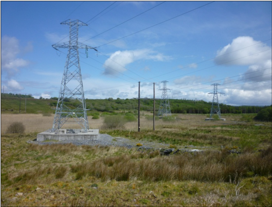
110kV angle towers at Srananagh Station with exposed substructures
