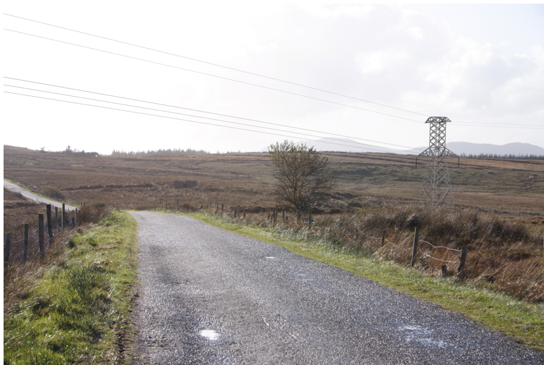
Figure 4.28 Example original ES Photomontage of Donegal 110kV line Reinforcement Project for ES Ref: viewpoint 2
