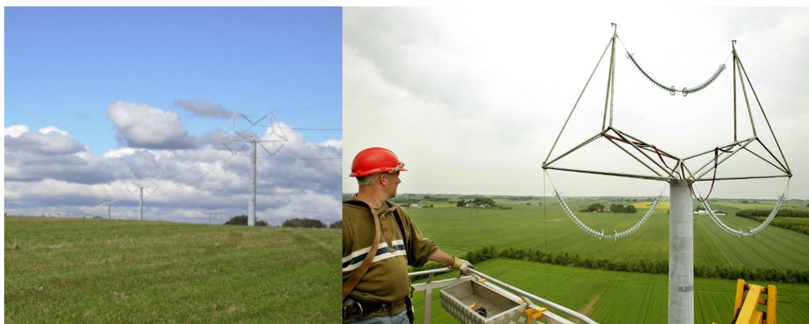
Figure 2.1: A new tower design for a 400 kV connection between the cities of Aarhus and Aalborg, Denmark (ENTSOE, 2012)
