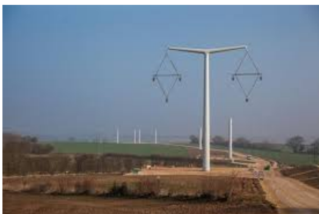
Figure 2.2: National Grid design competition winning “T-ylon” by Danish architects Bystrup on site (The Engineer Magazine April 2015)
