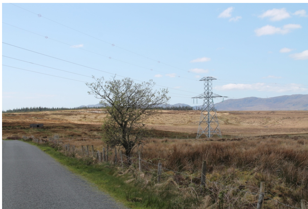
Figure 4.29 Photograph of “as built” Donegal 110kV line Reinforcement Project for ES Ref: viewpoint 2
