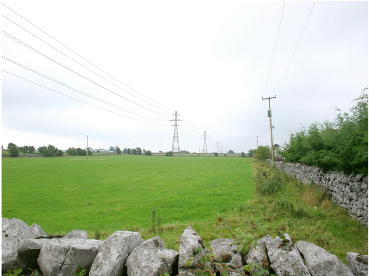
Figure 4.24 Example original ES photomontage (ES Ref: Viewpoint 1) Dalton to Galway 110kV double circuit line
