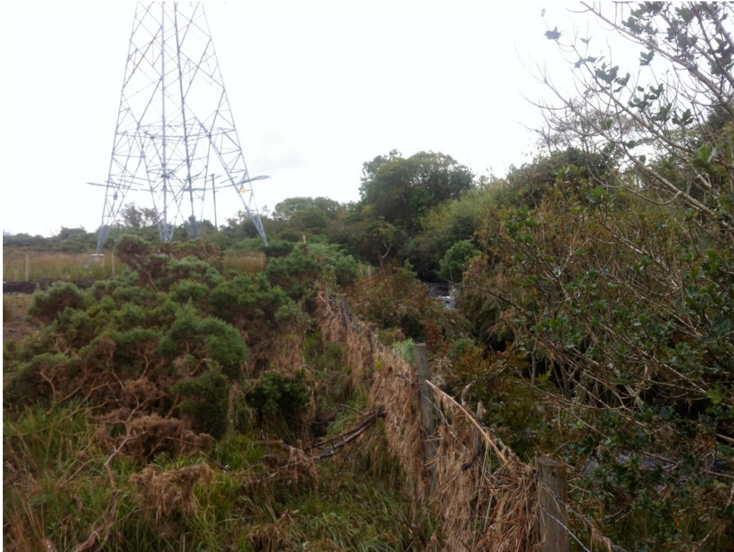
Plate 6.9 Image showing successful recovery of bankside vegetation and stability at AM196
