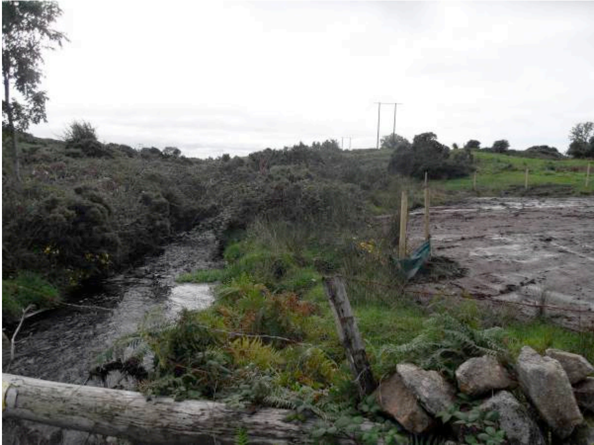
Plate 6.17 Site clearance works adjacent to the Barna Stream at AM9
