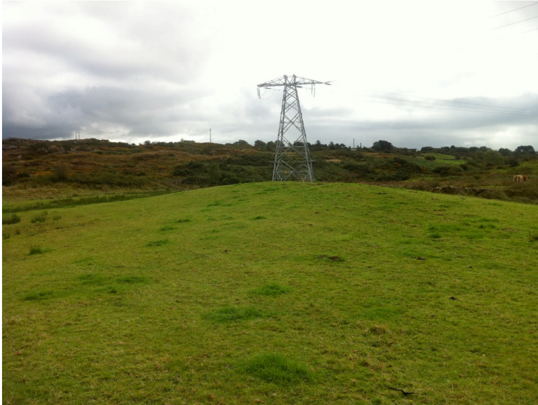
Plate 6.16 Evidence of complete recovery of field used for access during construction of AM9
