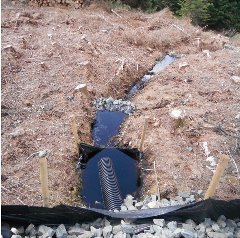
Plate 6.13 Silt curtains installed in drainage run-off from AM119
