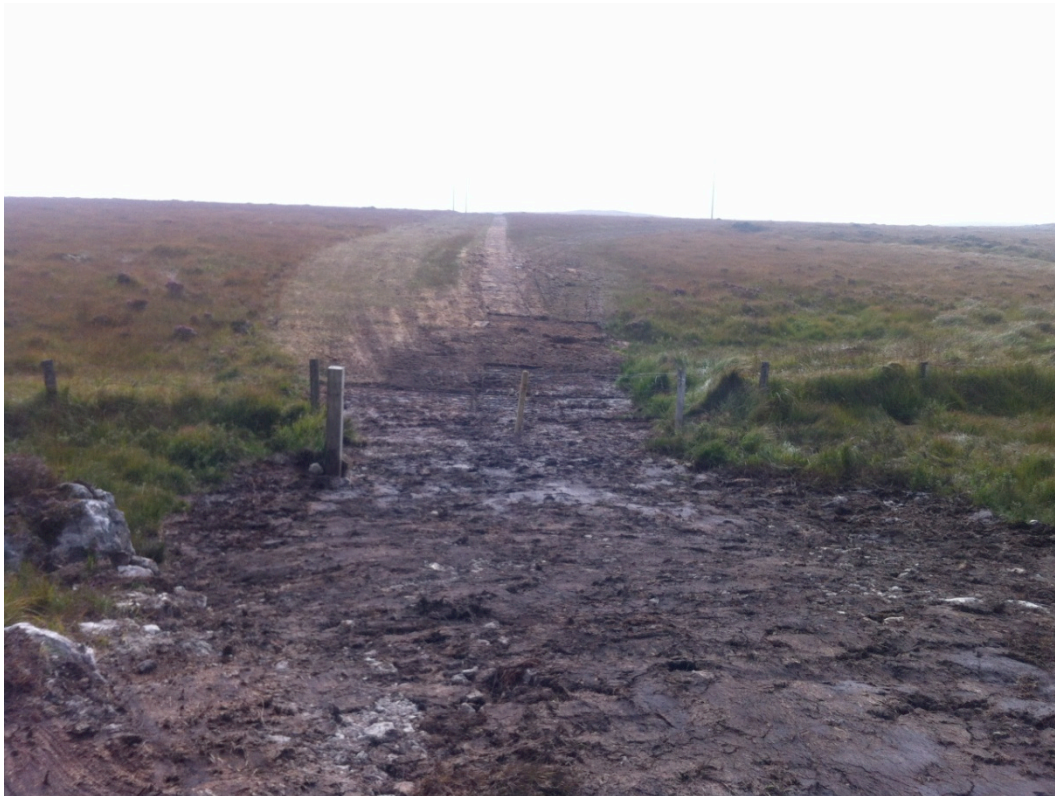
Plate 6.5 Ground disturbance during construction phase at AM173
