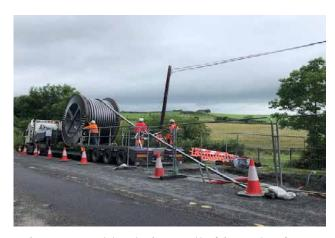
Figure 7: Cables being pulled into the ducts and jointing bay
