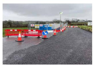
Figure 8: A typical passing bay in operation during cable jointing
