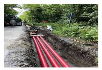
Figure 5: A typical cable duct installation in the road
