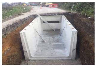
Figure 6: A typical jointing bay where cables are connected
