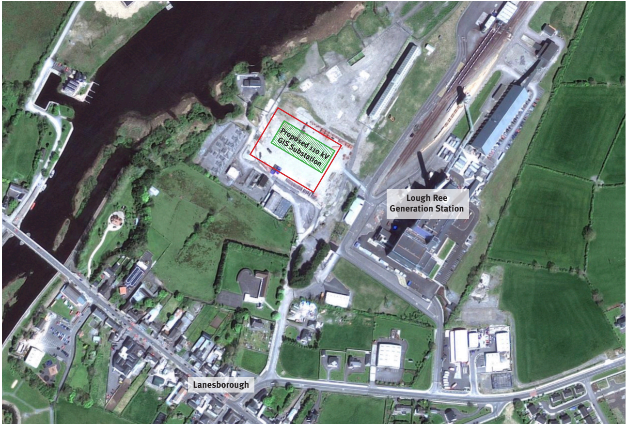
Lanesborough Substation Aerial View
