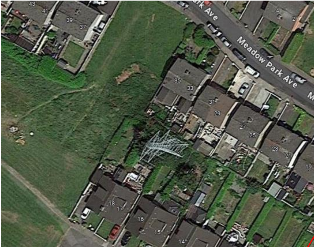
Kilbarry Marina 1 & 2 110 kV Double Circuit 27 th May 10 th September : 75 working days Partial refurbishment
