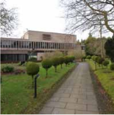
SONI Offices, Castlereagh House, Belfast.
