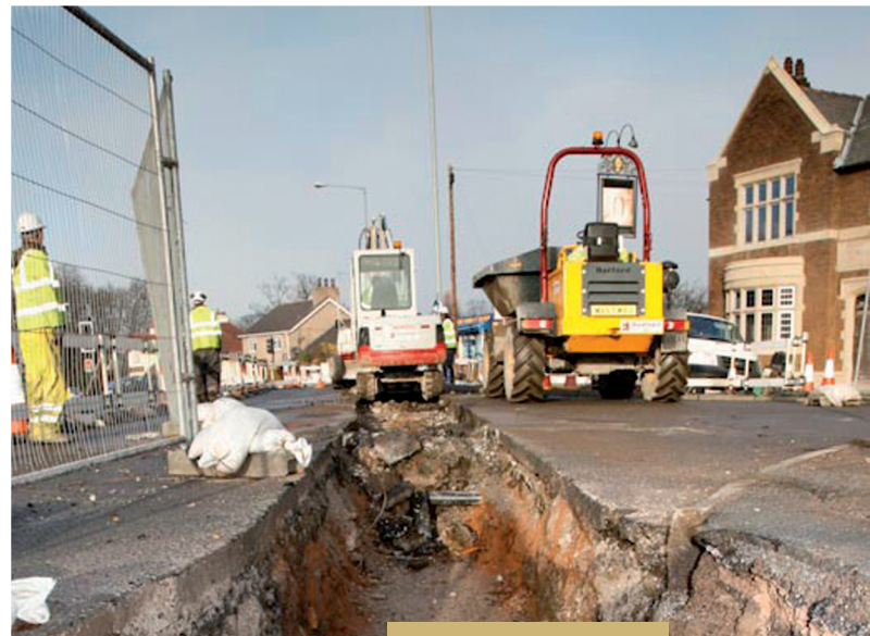
Construction work in Wales
