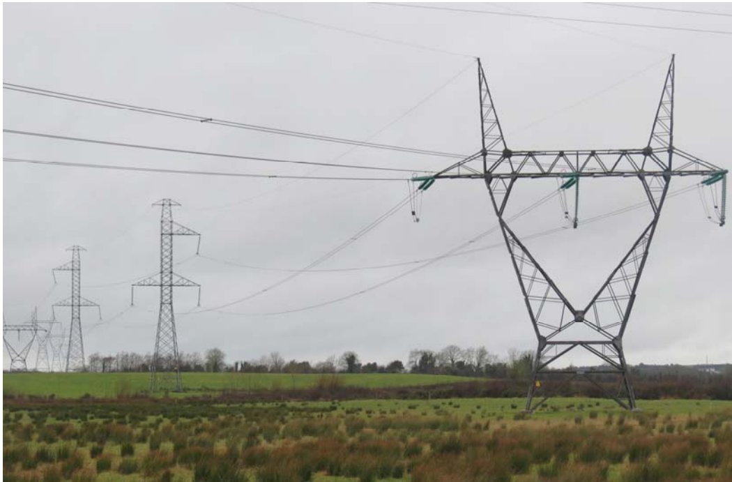
Photo 3: Transposition Alignment on an Existing 400 kV Overhead Line
